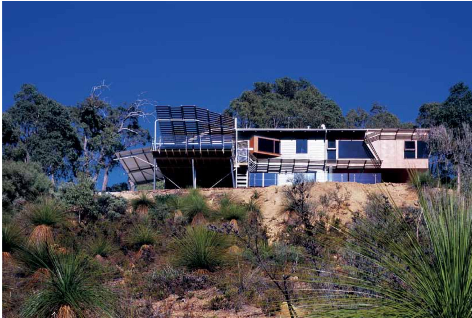
Upper level decks shade the rooms below, and the house is also protected from the harsh summer sun by a structure that encircles the house like a necklace. It's made of bent galvanised hollow-section poles and recycled jarrah timber, which formed the cladding on the original house
