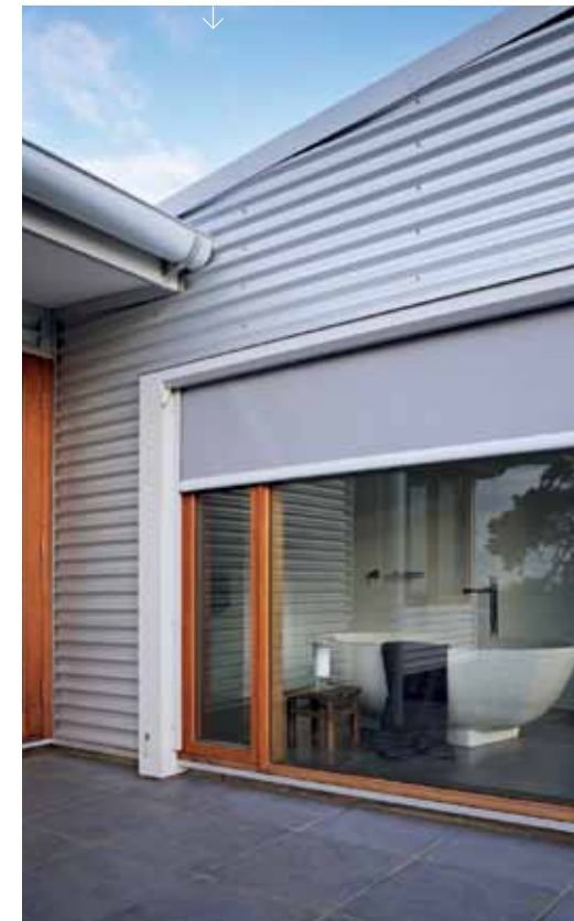
External blinds keep the summer heat from this north-facing room with a view
