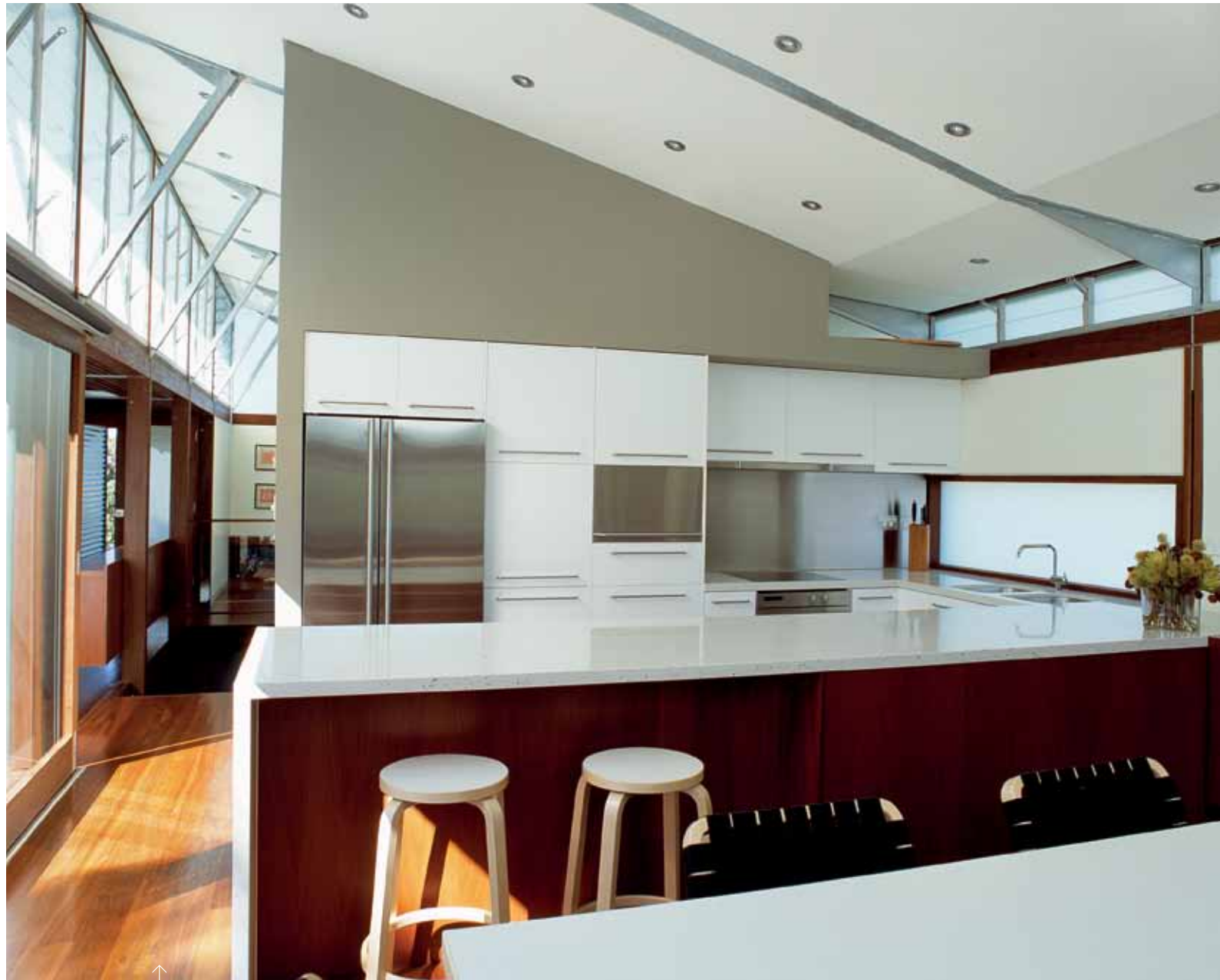
The floor is recycled ironbark, the structural frame, door and window frames are recycled jarrah
