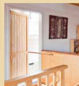
This home features two doorway-style cross ventilation features to capture cooling breezes
