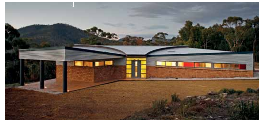
The compressed earth bricks on the southern entry side of house are a striking feature
