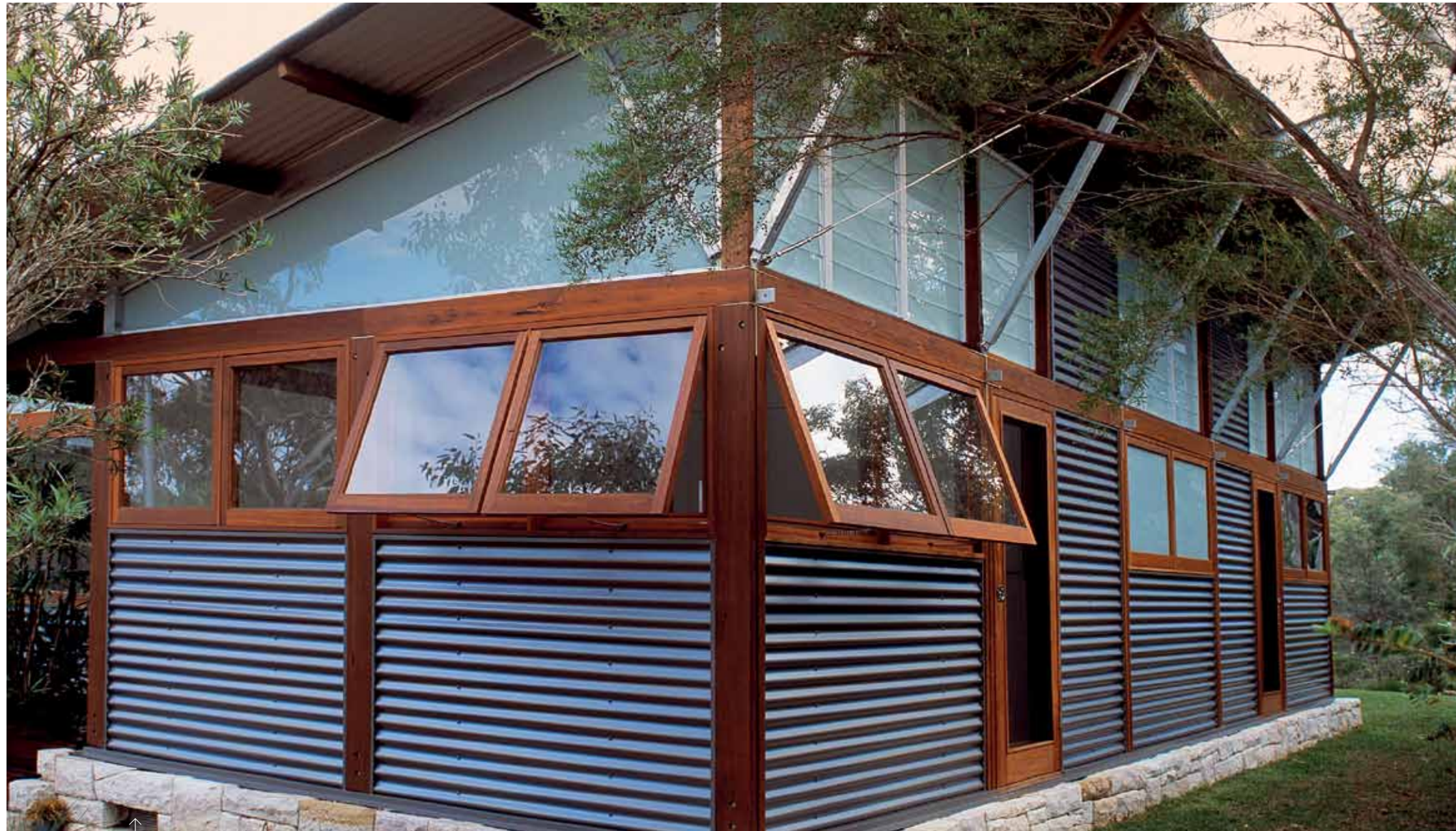
The pavilions are kept one room wide, to maximise light penetration and cross-ventilation
