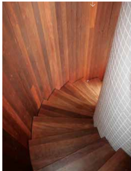
Stairwell comprises recycled brushbox reclaimed from a gymnasium
