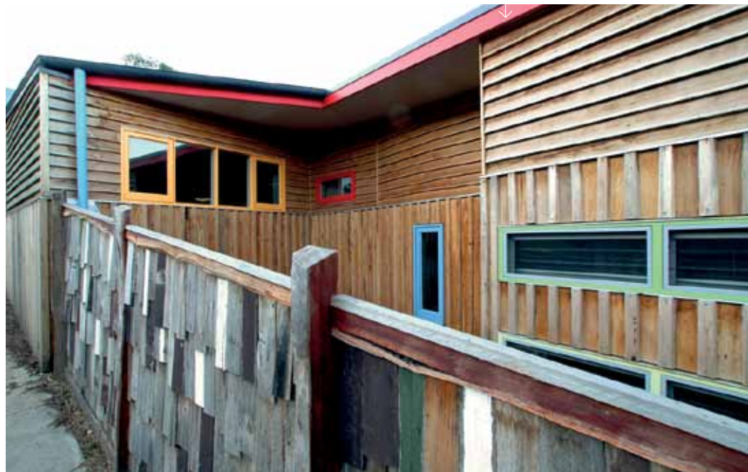
This fence comprises recycled old fence palings and railway sleeper cut offs
