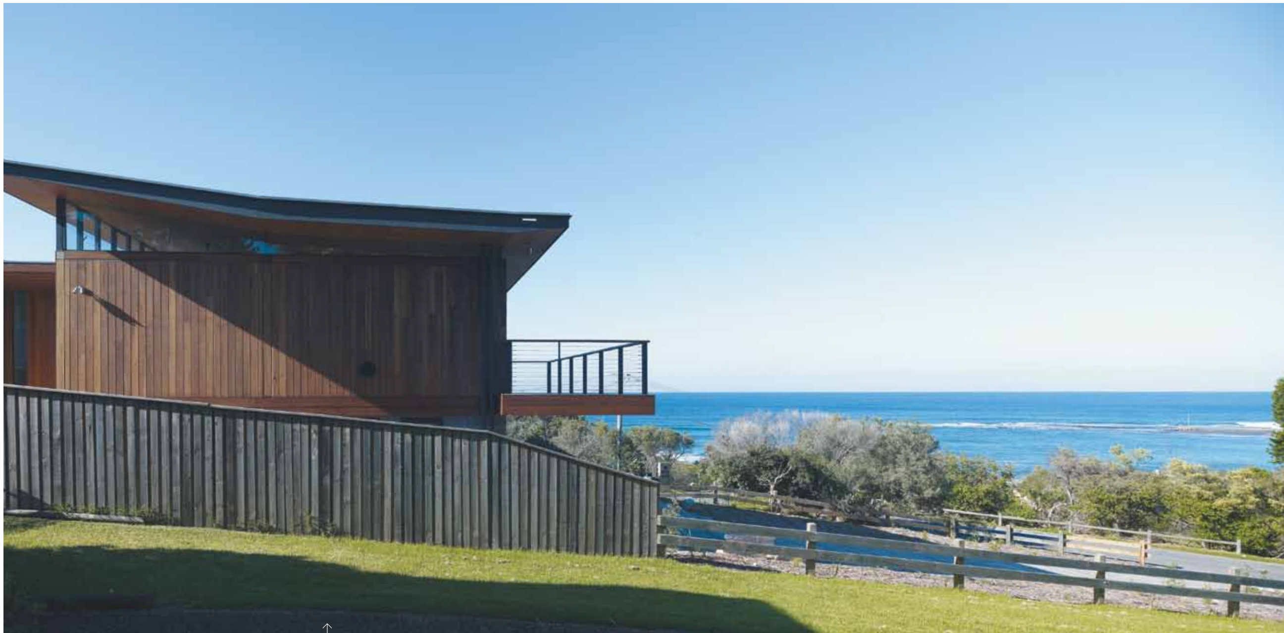
Shadowclad radiata pine eco cladding insulates reverse brick vener walls to the rear of the house
