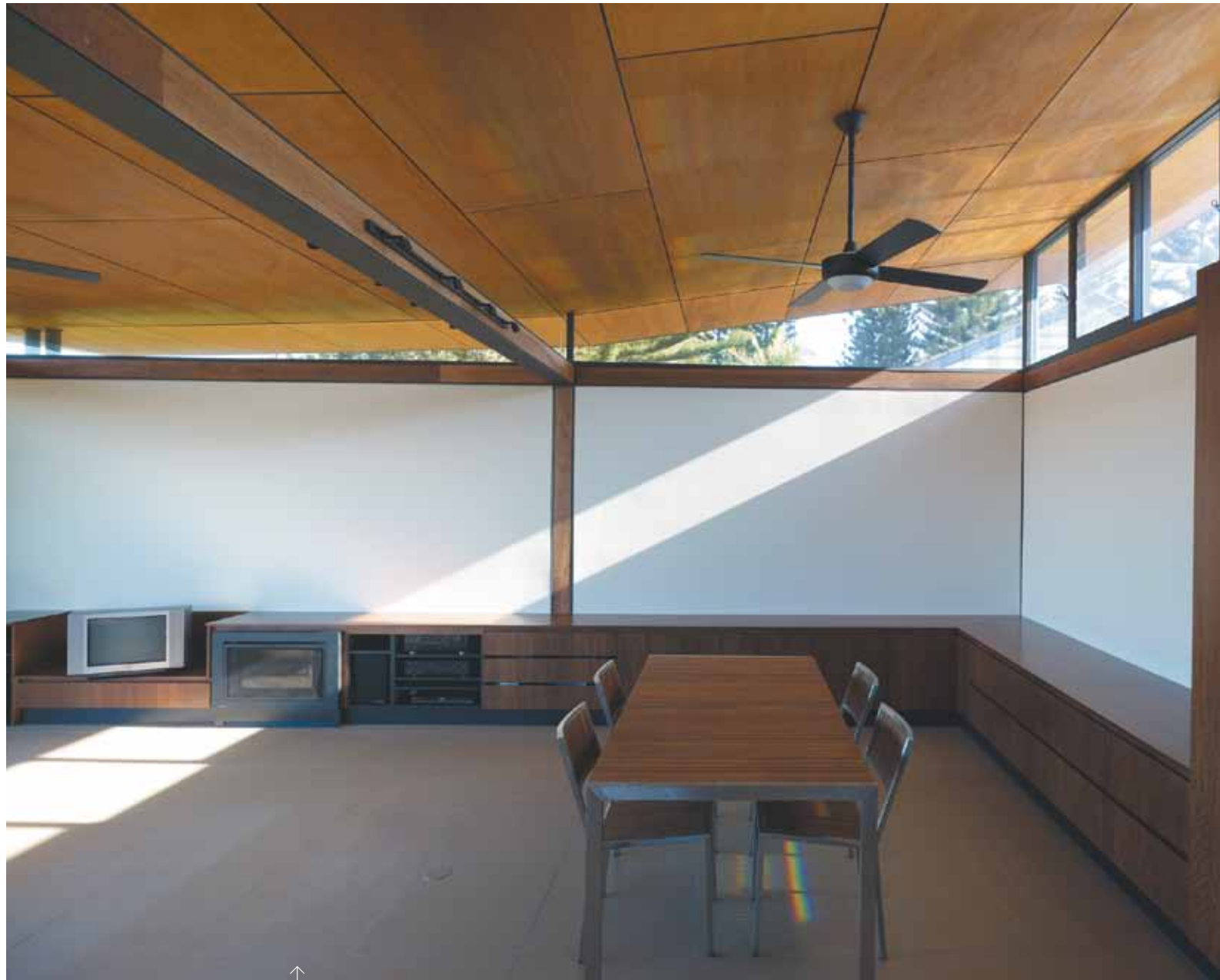
↑ Clerestory windows on the north wall of the south-facing living areas bring in light and warmth in winter. The rooms are also warmed by a solar hydronic system with pipes buried in the concrete floor, boosted by a high-efficiency gas heater
