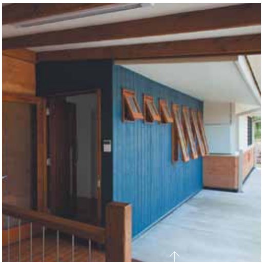
↑ Smaller openable windows on the south side minimise thermal loss while still permitting cross ventilation
