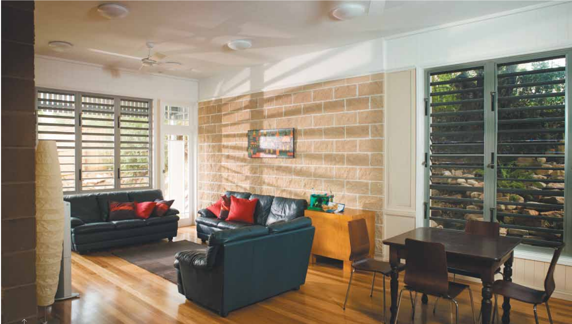
Reverse block veneer: The new addition stays true to the traditional Queenslander timber exterior but introduces a splitface concrete block wall to the interior for thermal mass, hugely improving the building’s thermal efficiency
