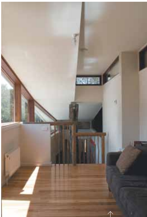
When the exterior door in this upper-floor room is opened, hot air rises from the ground floor through the stair void and is expelled
