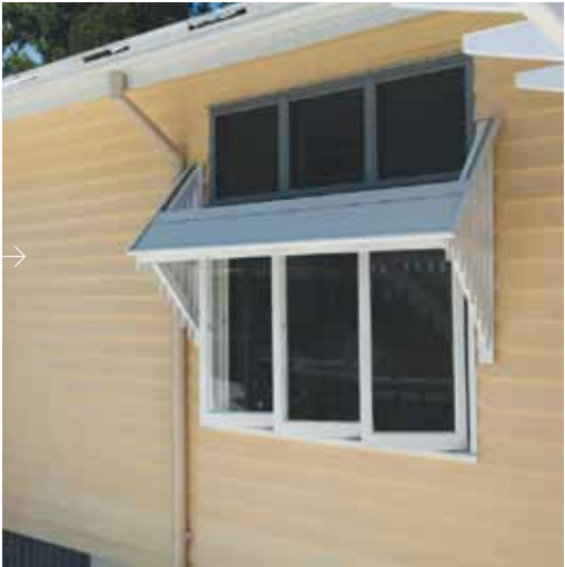
The original house awnings were modified and recycled
