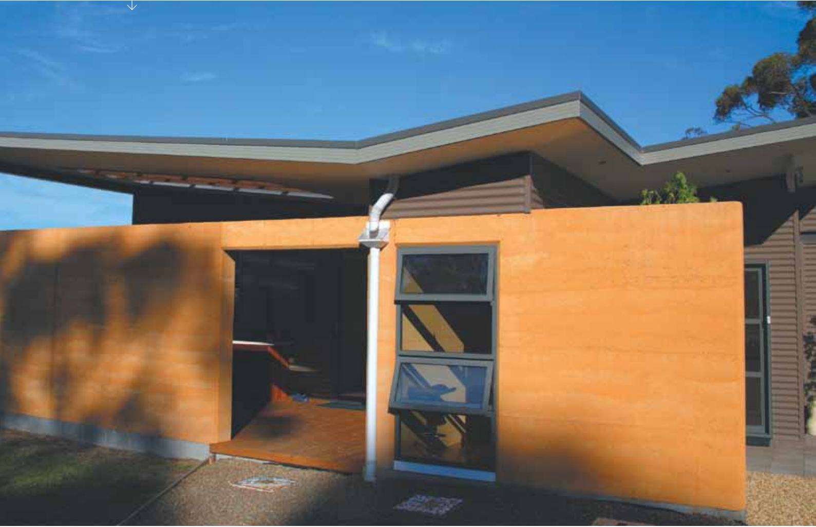
The butterfly roof funnels water to a central collection point, and down to five water tanks beneath the house
