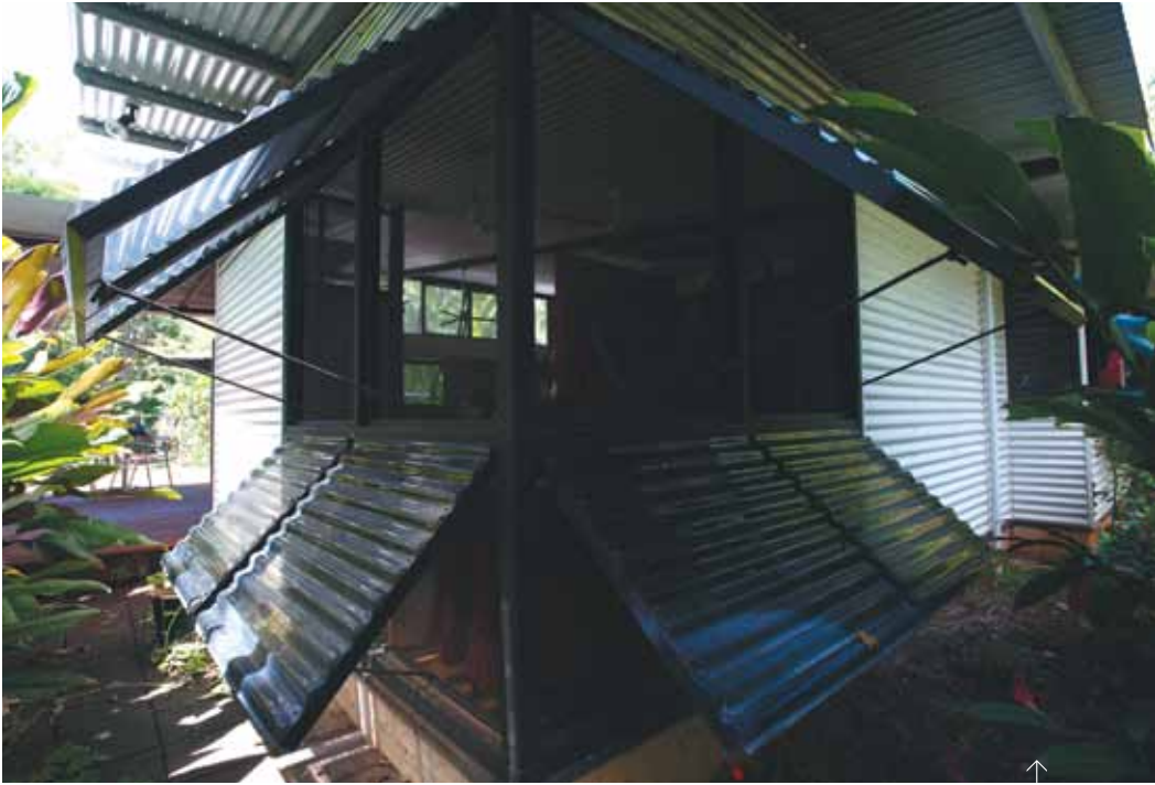
Awning shutters allow walls to remain open, even during tropical downpours
