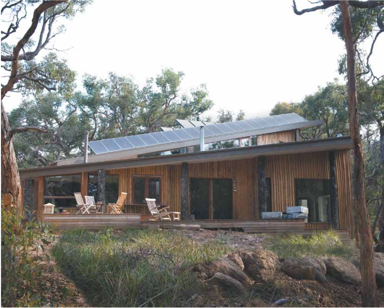
↑ The home's 3.3kW photovoltaic system is completely independent from the grid
