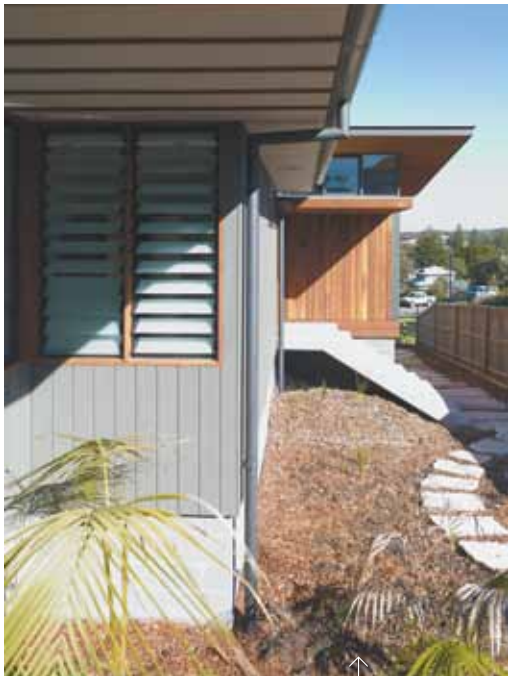
Bathroom exterior: louvered windows are positioned to provide good cross ventilation
