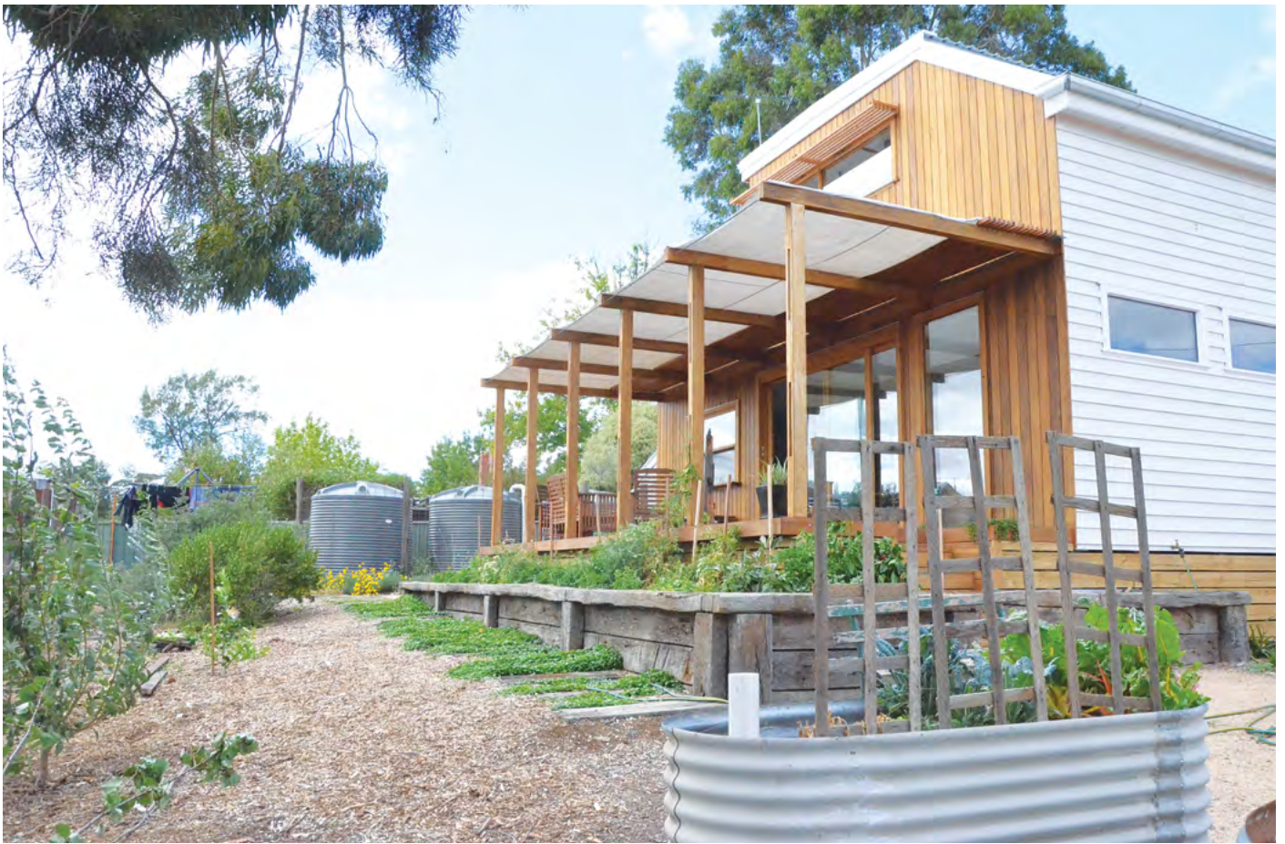
1 The modern northern addition and deck is clad in reclaimed blackbutt timber, and sits above recycled railway sleeper veggie planters. The mezzanine study and bedroom benefits from its own sunny balcony, a suggestion of Shae's. Temporary shading over the pergola will eventually be replaced by deciduous grapevines. The original bullnose iron roofing was used for wicking veggie beds.
