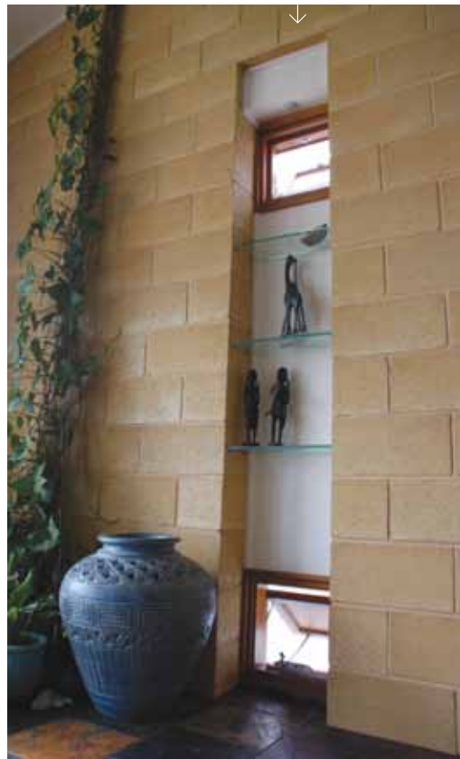
Passive-transfer hatches distributing heat from the glass house around the house
