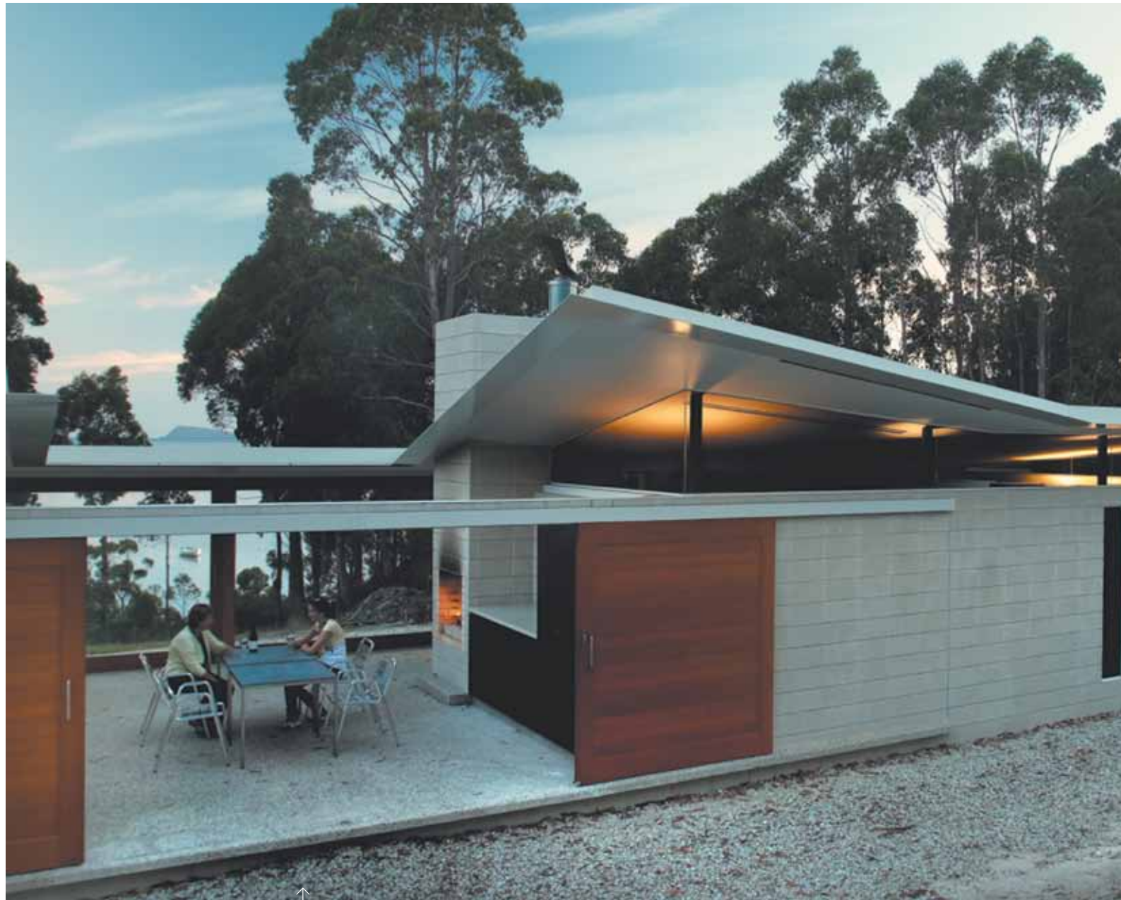
The aggregate used in the concrete floors was sourced from the site itself.
