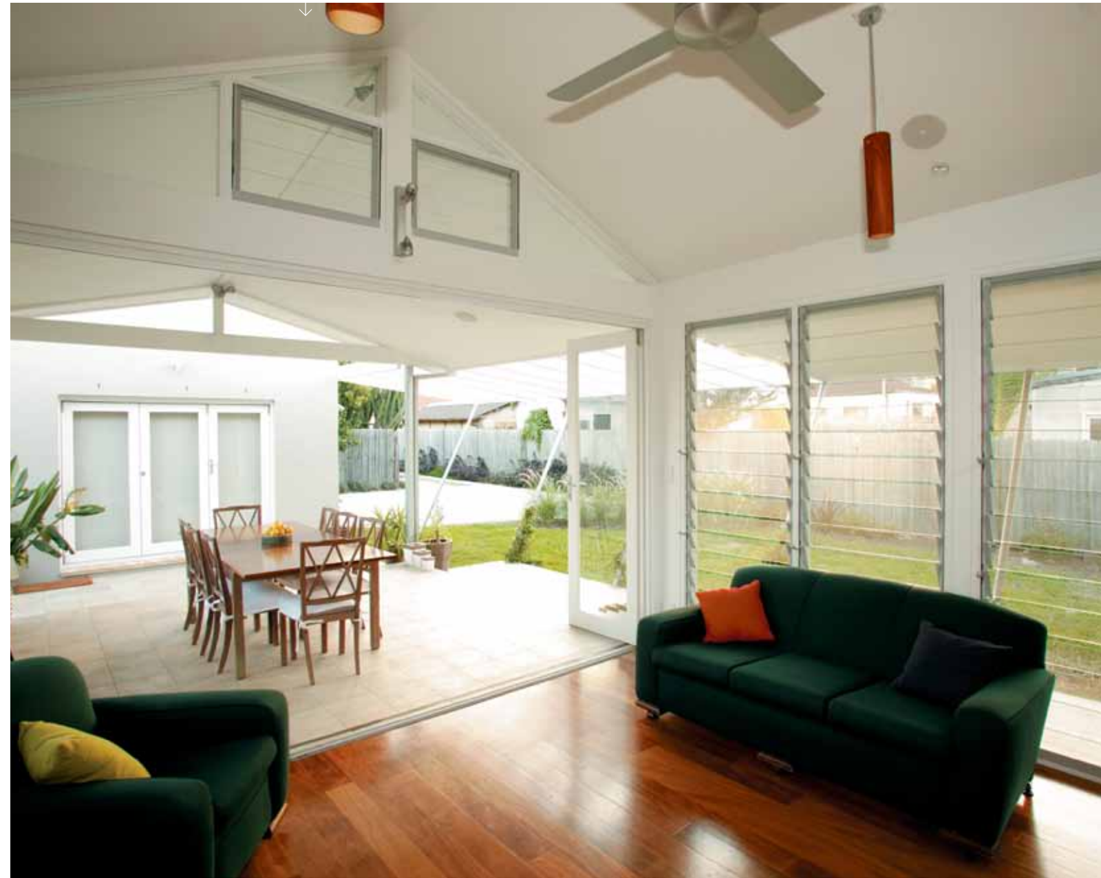
The new roof of the extension springs over the existing roof with glass louvres between the roof lines to allow air flow.
