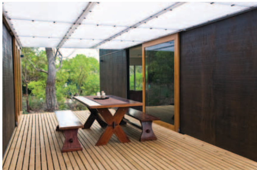
↑ Between the pavilions, the covered deck and its screening are made from eco pine and roofed with translucent acrylic.
