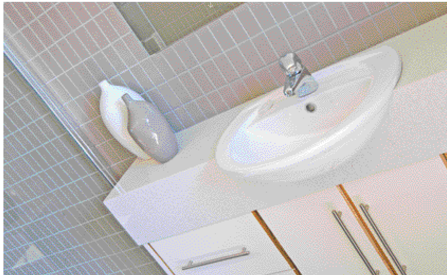
The bathrooms and laundry are fitted with AAA-rated taps and showers and the toilets are AAAA-rated dual flush units.
