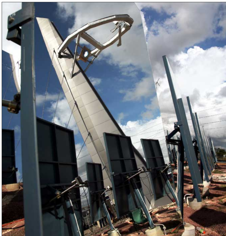
The 26 metre high solar tower that houses the solar concentrator is reflected in one of the 200 mirrors that help generate more than 500kW of power.
