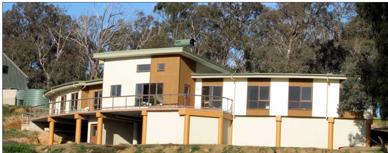
A passive solar home, packed with sustainable technologies in Melbourne's Green Wedge. Page 29.
