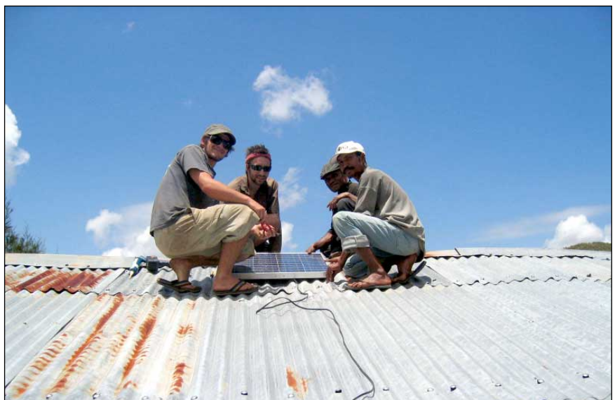
Installing a solar panel on a health clinic in the isolated enclave of Oecussi. This panel was capable of running six compact fluoros for up to four hours per night.
