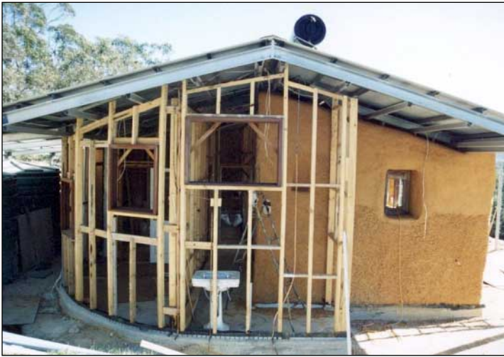
Above: Zoe applying some of the 40 tonnes of render to the outside walls. Top left: The in-slab floor heating system was installed before a concrete topping was poured over the existing shed slab. Left: The bathroom's stud walls before being 'baled'.
