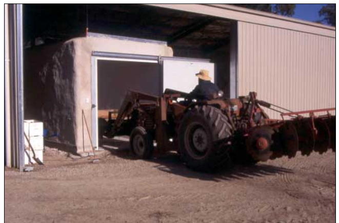
A bin full of organic pistachios are placed inside the strawbale cool room.
