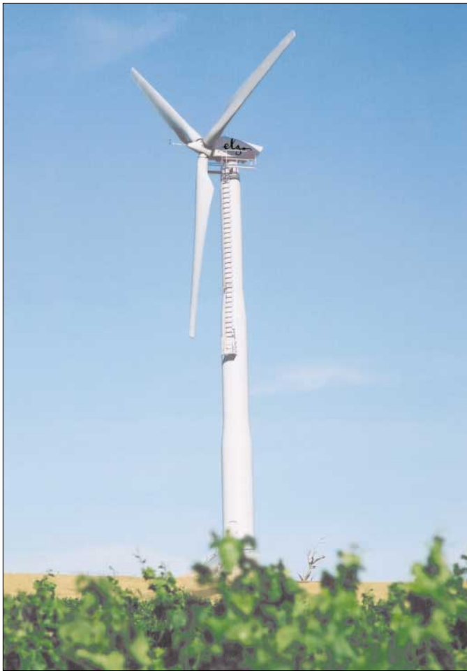
Wine gets a little help from wind—Elgo Estates' 150kW Bonus turbine set to go at their vineyard in the Strathbogie Ranges.
