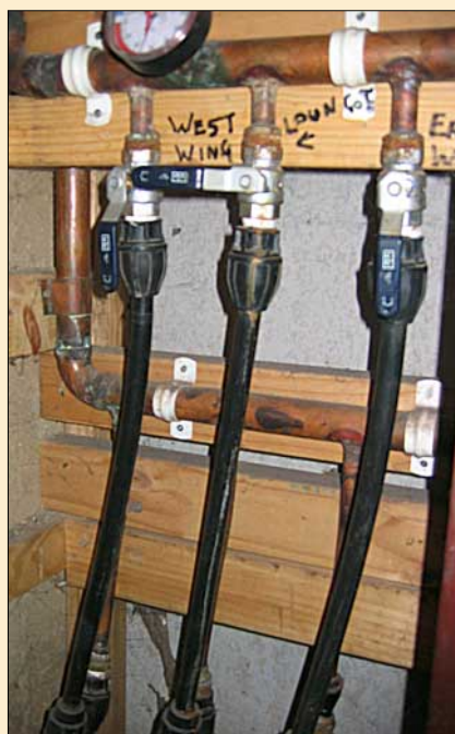
Multiple circuits in the hydronic heating system allow control over which rooms are heated.
