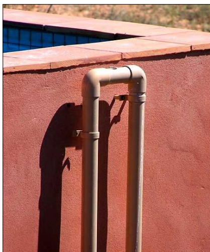
A breather in the overflow pipe was needed to stop the siphon effect from emptying the pool!
