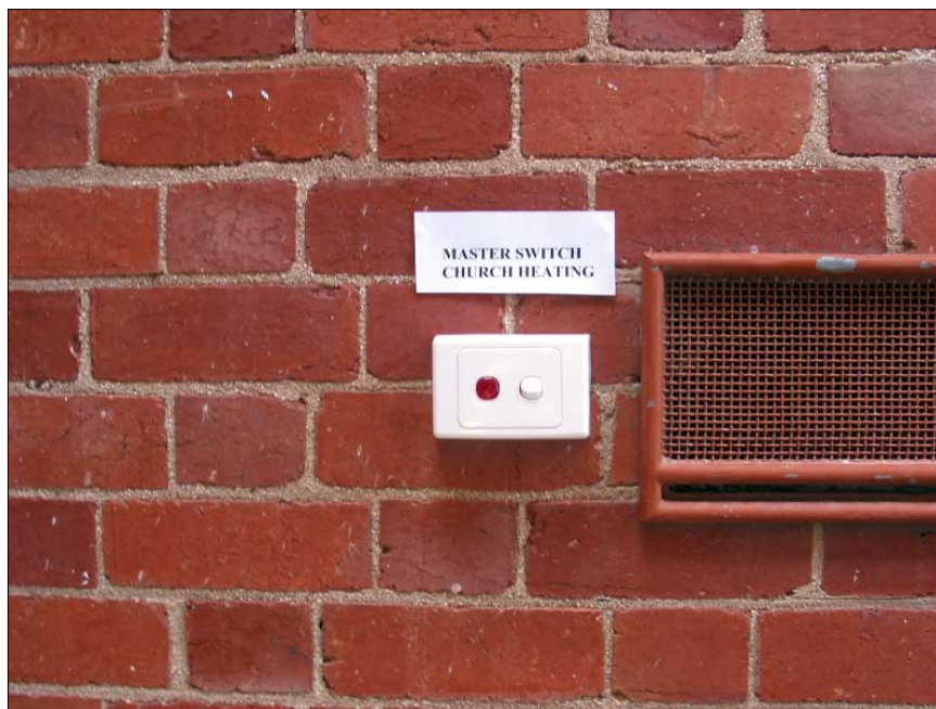
The master switch installed at Ivanhoe Uniting Church turns off all the heaters in one go!
