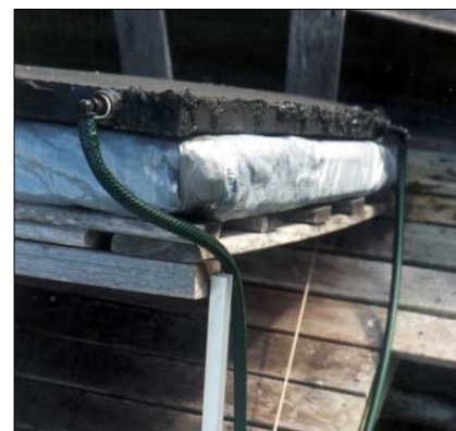
Closeup showing the collector panel on top of the frame, with the insulation pack between them.
