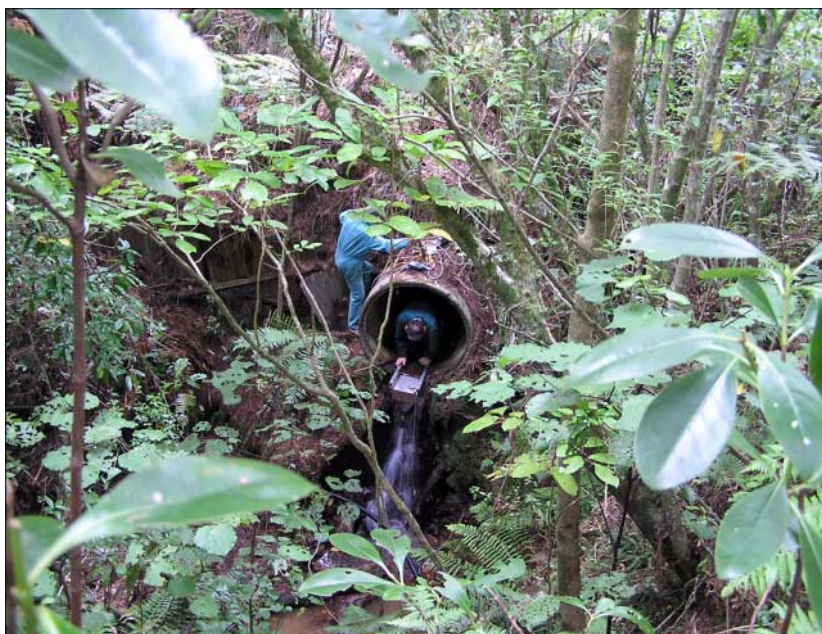
Left: The intake screen is positioned in the culvert, excess water flows over the screen keeping it free of leaves and other debris. Right: Everbody lends a hand to help install the piping.
