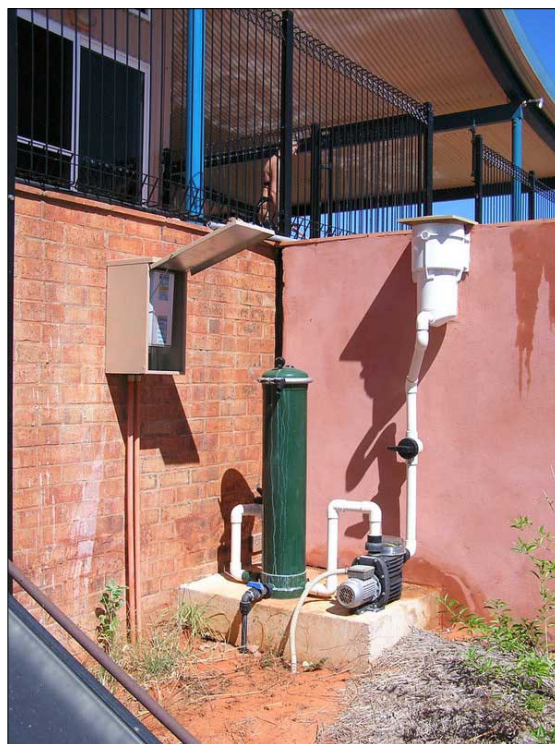
The MPPT and pump system for the swimming pool.
