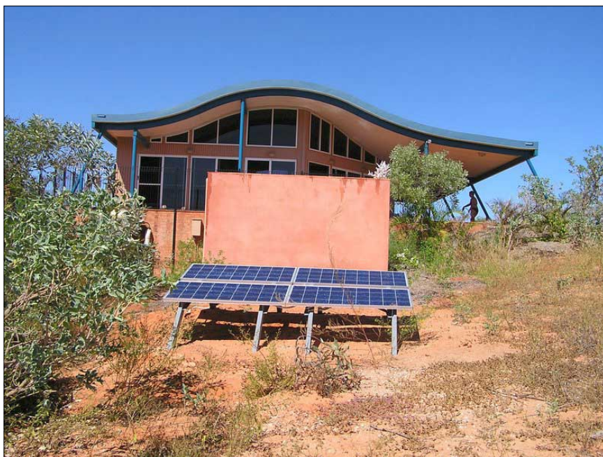
This solar array is all that was needed to run the pool-pumping system.
