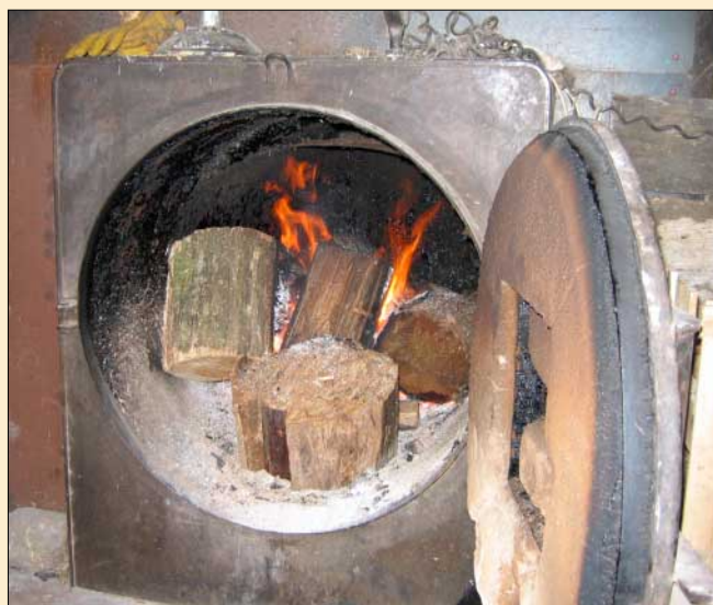
The boiler's firebox can use as little as two logs, or as much as three barrow fulls of wood per day, depending on the season.
