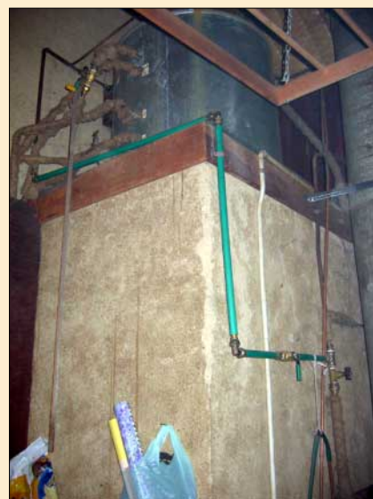
The hot water storage tank.
