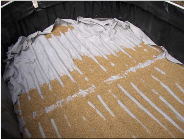
Laying the gravel filter in the bottom of the pool.
