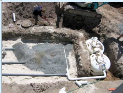
6. Pipes distribute greywater over the total area.
