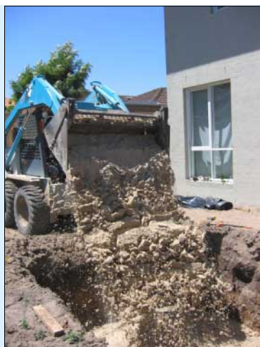
2. Filling sand filter—first layer.
