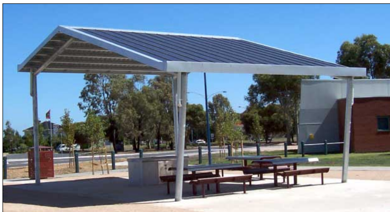
The solar panels on the roof of the shelter supply power for the bbq.
