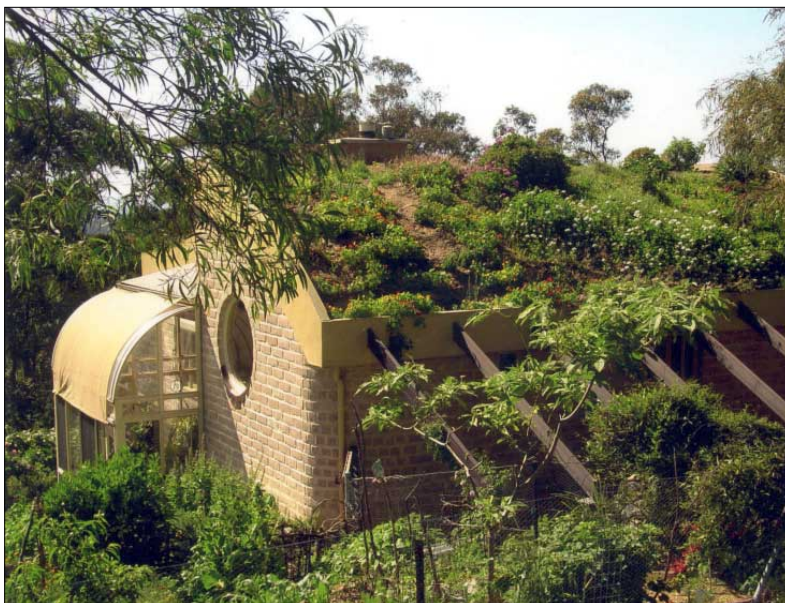
Blue Mountains retreat: a mudbrick house with an earth-covered roof. Page 23.
