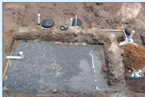
7. The sand filter system is complete and ready to be covered by lawn.
