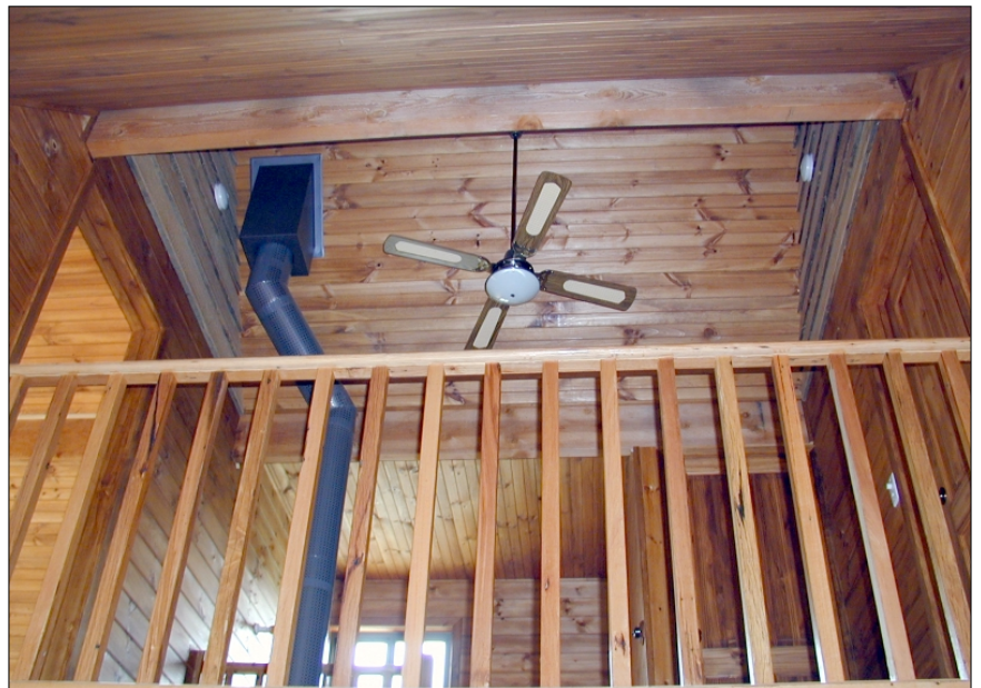
Radial cut native timber was used for the roof, and the upstairs exterior and interior walls.
