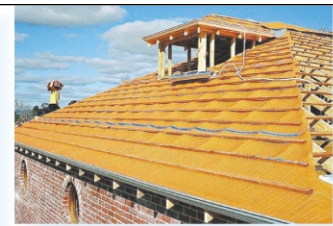
AIR-CELL Insulation delivered both a sarking and a 4 star energy rating when installed under this tiled roof.
