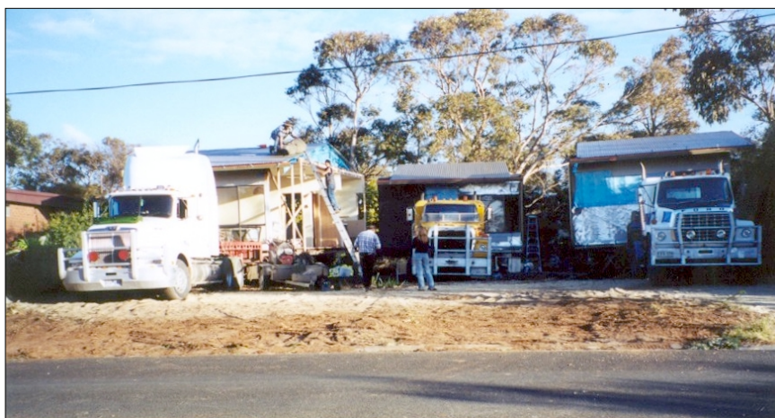
The house divided into three trailer loads and ready to hit the road.
