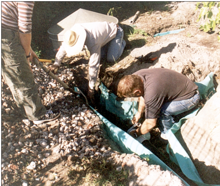
Left: Workshop participants place the aggregate in the geotextile-lined trenches.
