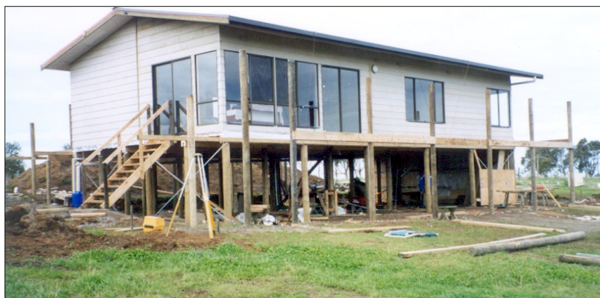
The relocated house, elevated and in the process of being 'decked' out.
