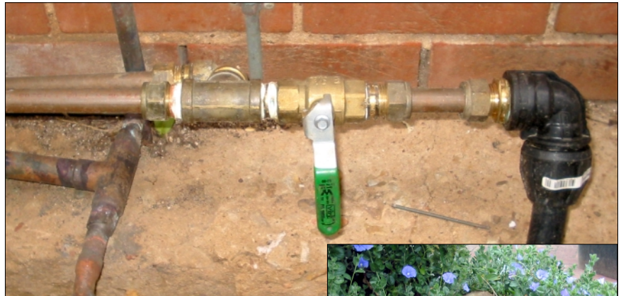
Above: The pressure pump is connected to the closest 19mm mains line.
