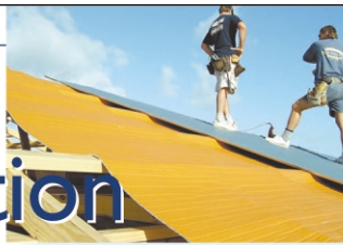
AIR-CELL Insulation directly under this conventional metal roof provides R_{t2.5+} installed performance.
