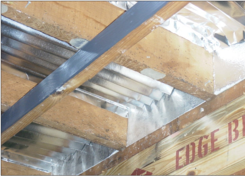
Insulation, like these foil batts, is very important in keeping a house at a livable temperature.
