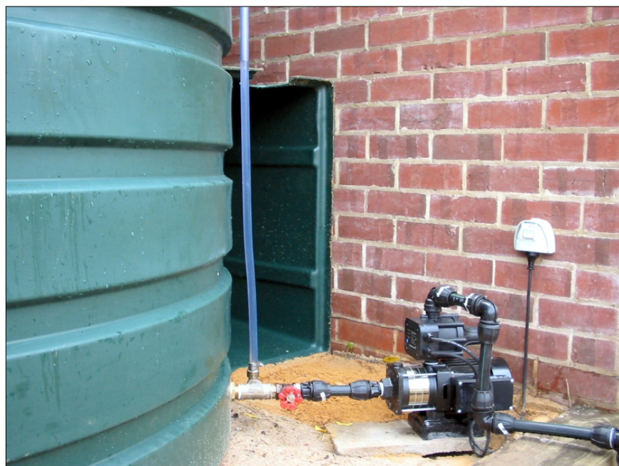
The rainwater is fed into the home's water piping by the use of a pump.
