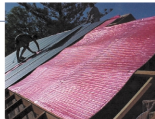
AIR-CELL Insulation directly under this conventional metal roof provides R t 2.5+ installed performance.
