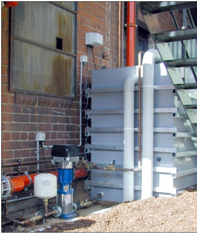
Left: The new rainwater tank that feeds water to the toilets for flushing.
