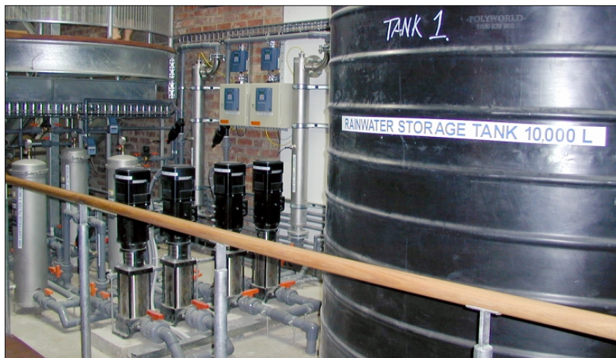
The water from two 10,000 litre rainwater tanks is treated via the filtering system at left and supplies the drinking and shower water for 60L. Greywater from the on-site biological sewage treatment system is used for toilet flushing and on the gardens.
