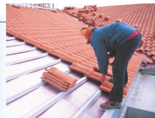
AIR-CELL Insulation delivers both a sarking and a 4 star energy rating when installed under this tiled roof in WA.
