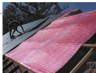
AIR-CELL Insulation directly under this conventional metal roof provides R2.5+ installed performance.
