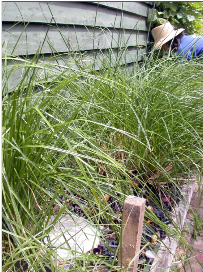
Water from the bathroom filters through this reed bed system (made from objects reclaimed from landfill) and is used to irrigate the garden.
