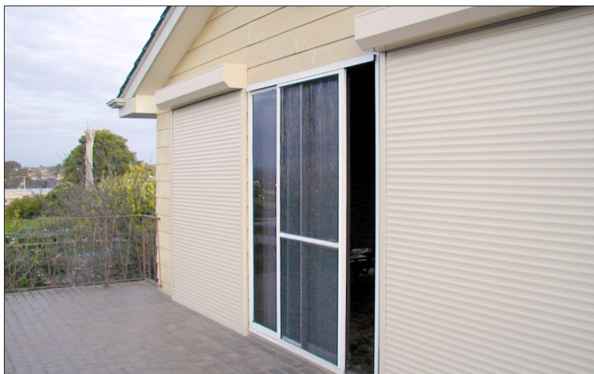
Before these roller shutters were installed, this upstairs, north-facing, room was unbearable in summer, yet pleasant in winter — now it can be used year-round.
