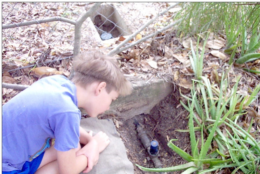
Here the dual check valve and pressure reducing valve (and Dave's son Hunter) can be seen. The council water meter and stopcock are just on the other side of the fence.
