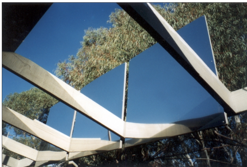
Derek installed three highly-polished sheets of stainless steel outside of two south facing windows to reflect more light into his home.
