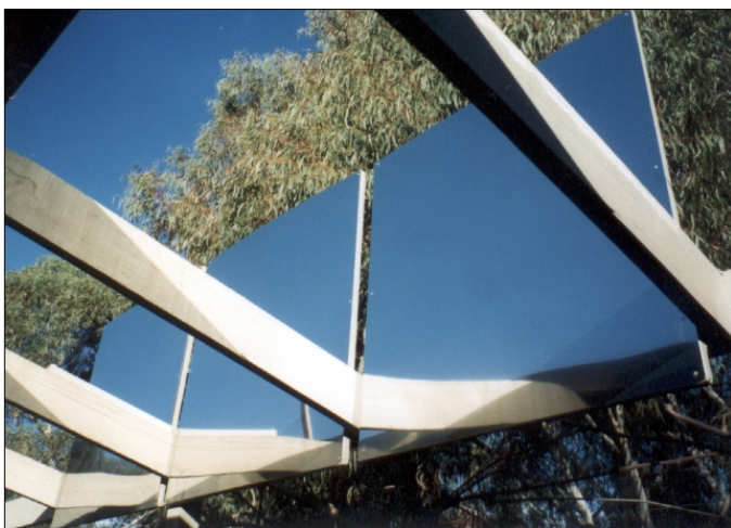
Left: These polished stainless steel solar reflectors are one retrofitter's method for ensuring the south-facing rooms of his home receive sunlight year-round. Page 21.
