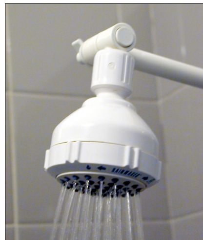
Low flow shower heads not only save a lot of water, but the energy used to heat it as well. This unit is an Interbath Rainmaker.
