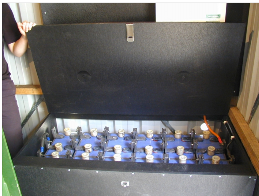
The battery box and battery bank. The recycled plastic board makes for a nice finish to the job, and is completely acid proof, unlike wooden boxes. Stainless steel connecting bolts and box hinges are also a must, as are the vents, visible at the top corners of the rear of the enclosure.
