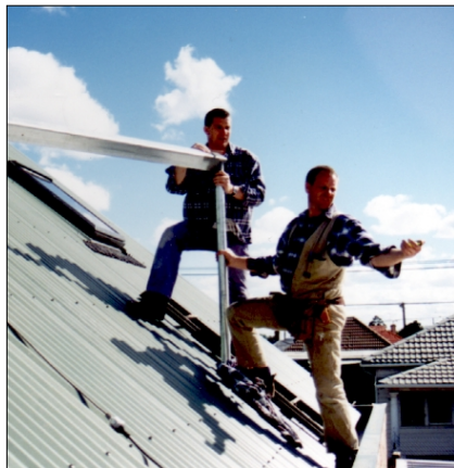
Roger uses a compass to ensure his solar water heater faces due north.
