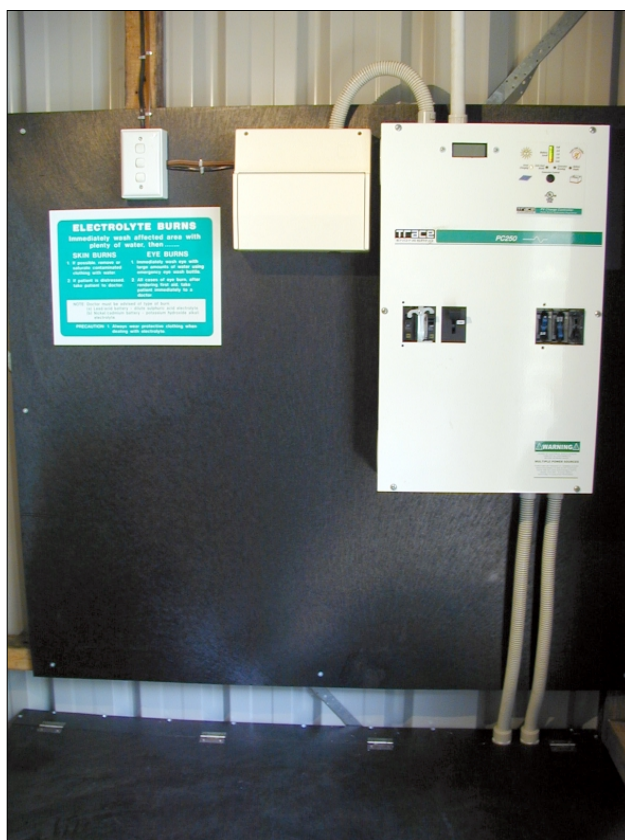
The Trace PC250 controller (on the right) mounted above the battery box on another sheet of plastic board. The smaller box to the left is the DC load circuit breaker box. Also note the safety sign on the left, placed to be easily visible.
