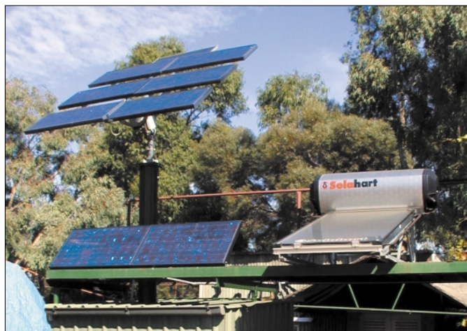
New additions to the ReNew and ATA power system.
