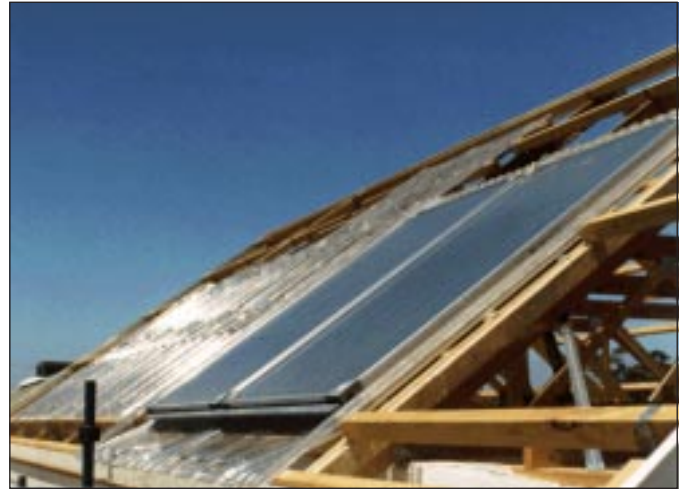
Left: The SolarSense home complete with Solar Energy Roof. Right: The Roof integrates photovoltaic cells, a skylight and solar water heating panels into one panel. The solar componentry is fitted into a plastic tray that is laid on battens before the colourbond roof. Note the 'shoe' to the drain for the solar heater.
