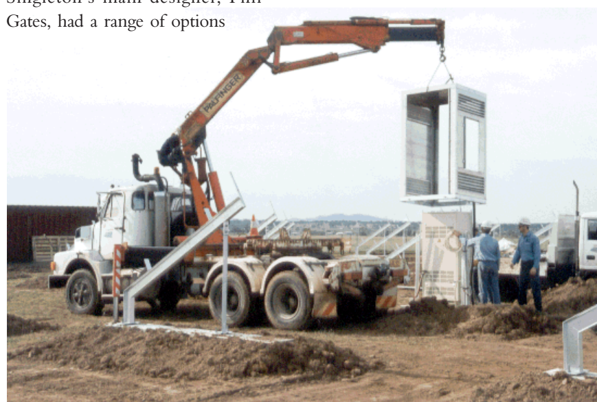
Installing a cover for a Power Solutions inverter at Singleton.
