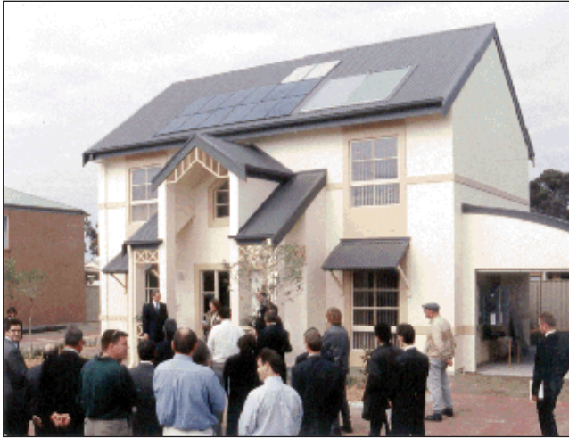
Left: The SolarSense home complete with Solar Energy Roof. Right: The Roof integrates photovoltaic cells, a skylight and solar water heating panels into one panel. The solar componentry is fitted into a plastic tray that is laid on battens before the colourbond roof. Note the 'shoe' to the drain for the solar heater.
