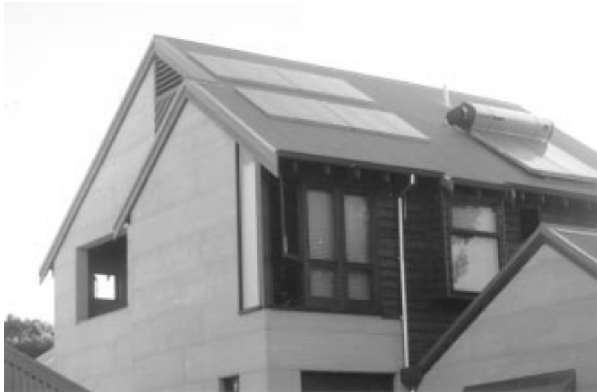
Bill's house uses the electricity grid like a battery, feeding in excess solar energy from the photovoltaic panels (left) and drawing it back as needed during the night. Hot water is provided by a Solahart solar water heater (right).
