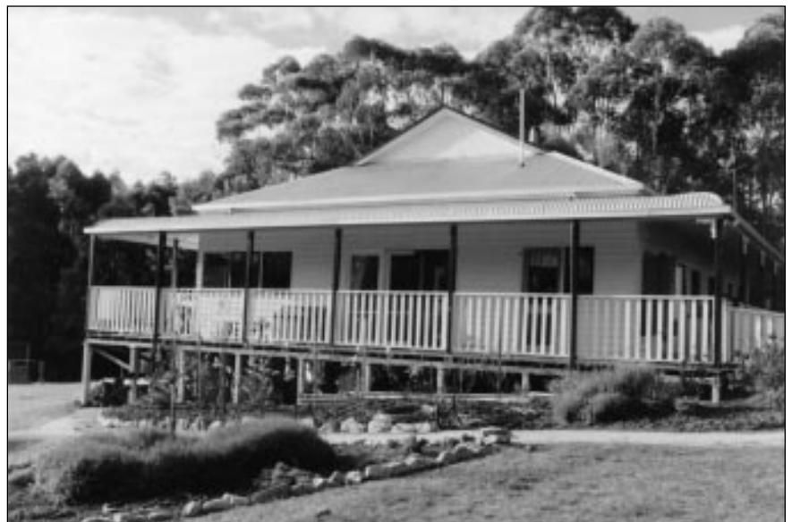
The house is a Federation-style weatherboard. The bull-nosed verandah is designed to be high enough to allow natural light in, while still shading the house in summer.
