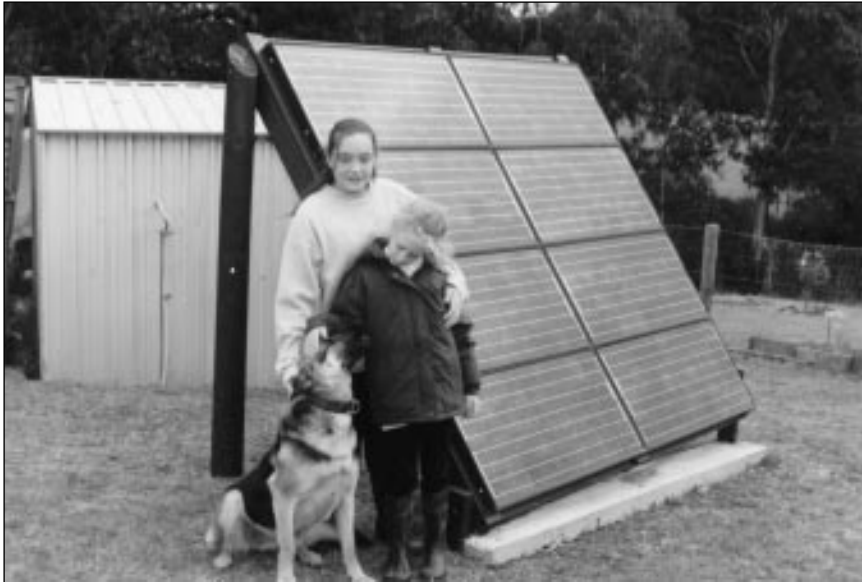
Lauren and Stephie both agree: the solar panels are very pretty, especially in full sunlight. The frame can be tilted to optimise power from summer and winter sun, and a concrete strip protects them from mowers and wipper snippers.
