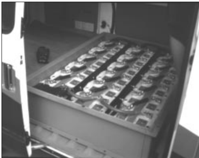
Here you can see the bank of Optima YellowTop batteries. There are 18 Optimas providing 72 volts to the series wound DC motor via a 400 amp controller.
