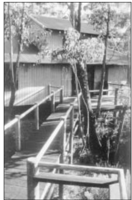
The walkways at Jemby Rinjah Lodge limit movement through the bush, while still allowing viewing access and the feeling of being a part of it, and also keep all the human traffic above the ground so that plant-life and fauna is not disturbed.
