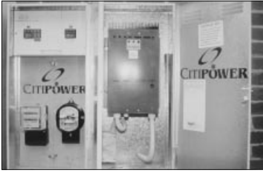
Above: The house has two electricity meters—one for billing and one for measuring output from the solar panels. The CSA inverter is to the right of the meters.
