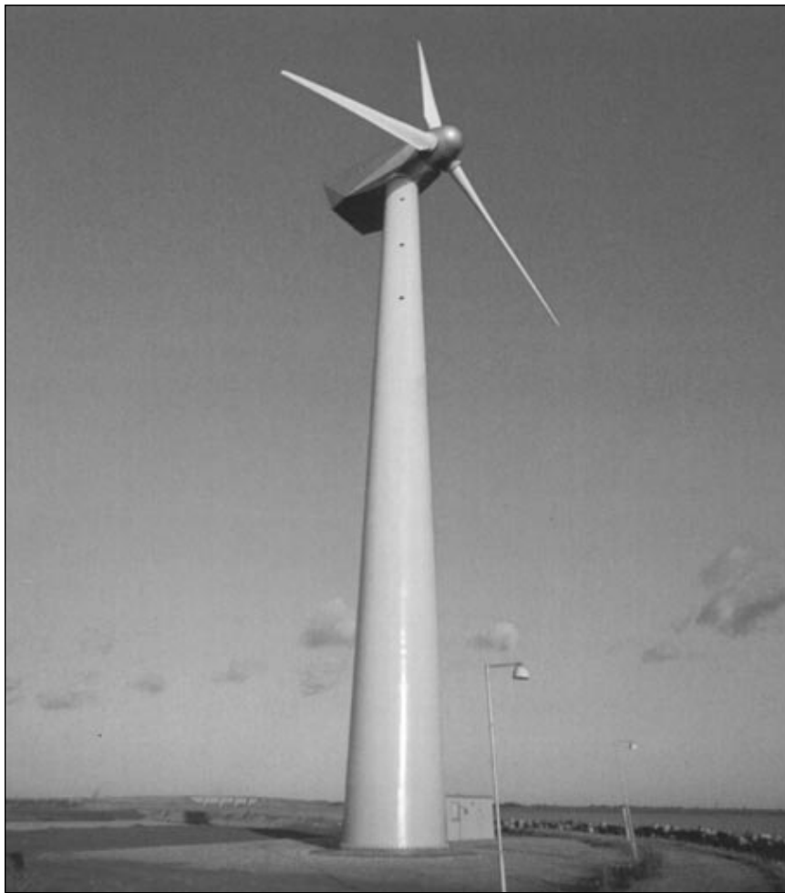
A 1 megawatt wind turbine at Avedøre Holme, south of Copenhagen, Denmark.
