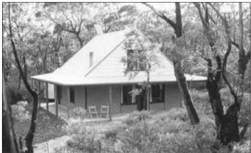
The Bungaree Cottages in the Blue Mountains use mudbricks for thermal mass and solar panels for electricity generation.
