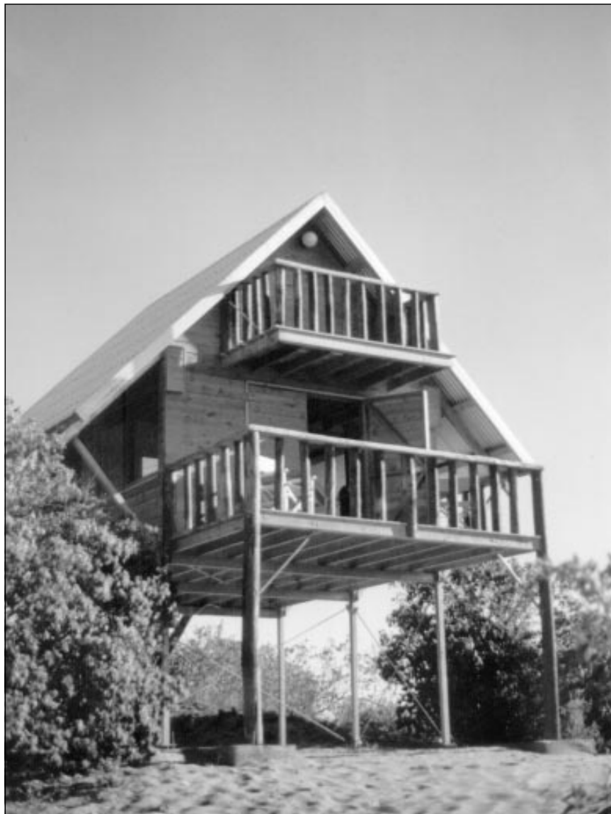
One of the passive solar huts at Eco Beach resort. Smart architecture saves the owners of this resort between $15,000 and $30,000 per year on air conditioning running costs.
