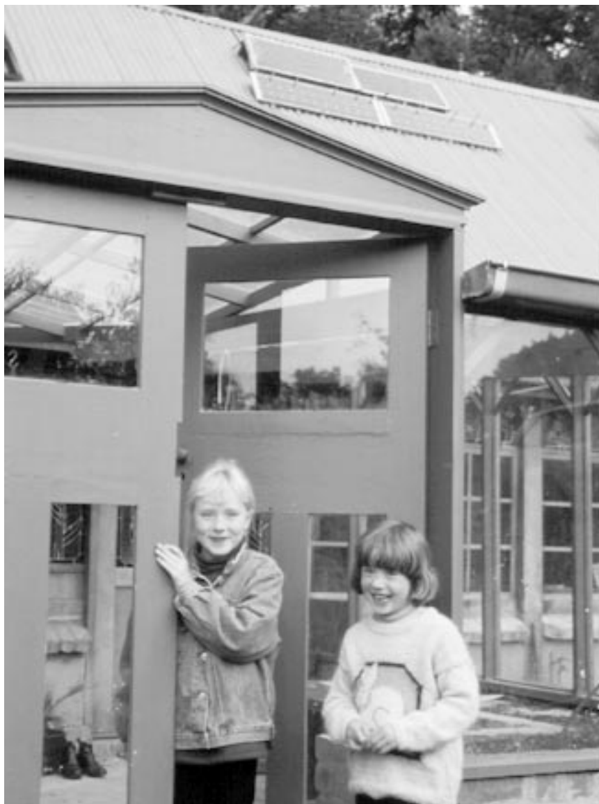
Cover models: Linden (left) and Tessa Smith in front of their solar powered house at Moora Moora. The glassed entrance area traps sunlight to provide free heating for the house, as well as creating an airlock between the front door and the often cold air outside.
