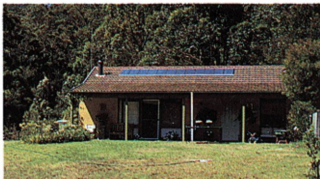
Off grid solar/diesel hybrid system
