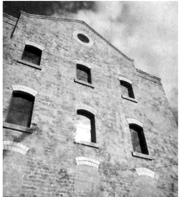
Shugg double-hung sashless windows provide ventilation through the top and bottom of the window.
