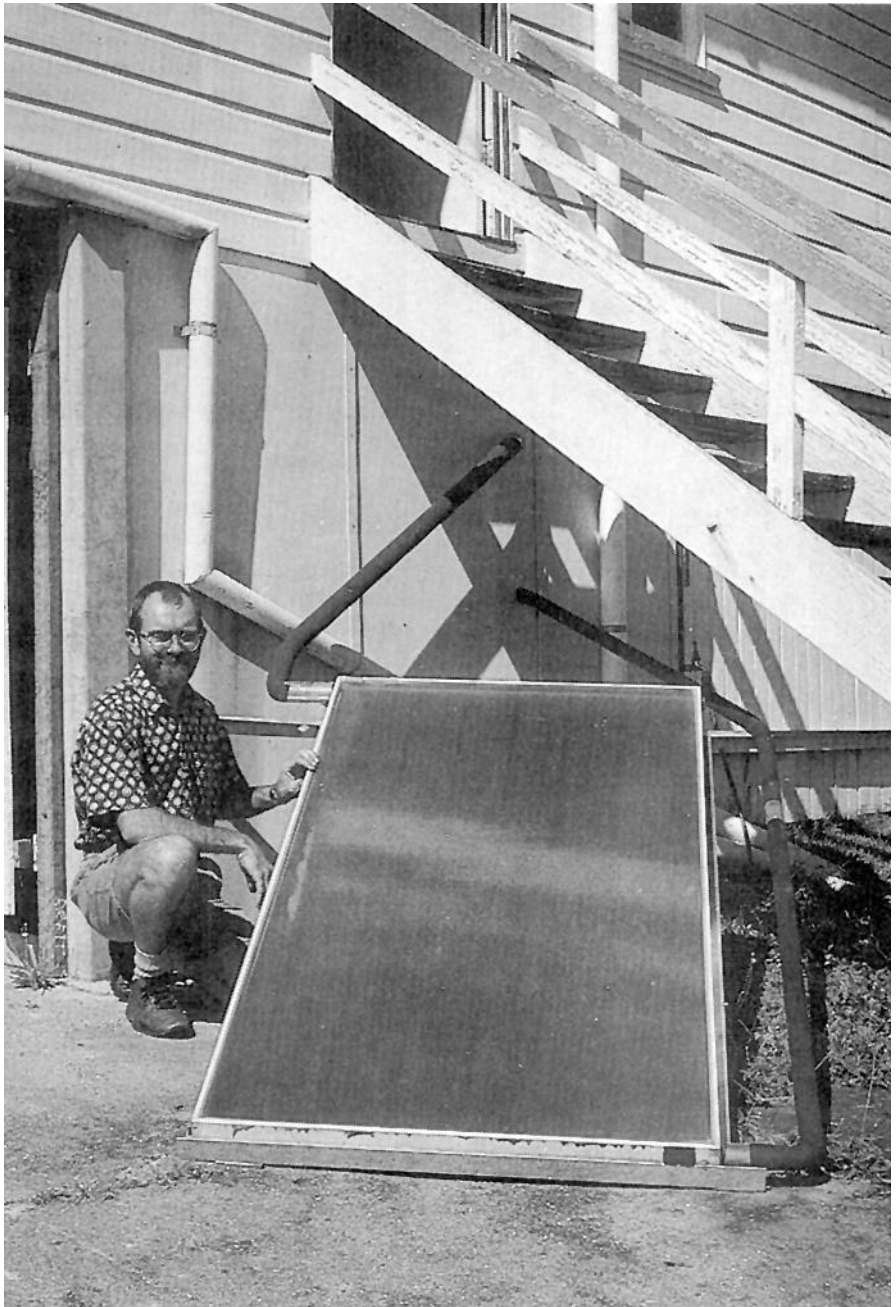
Trevor with the solar collector mounted on the western side of his house.
