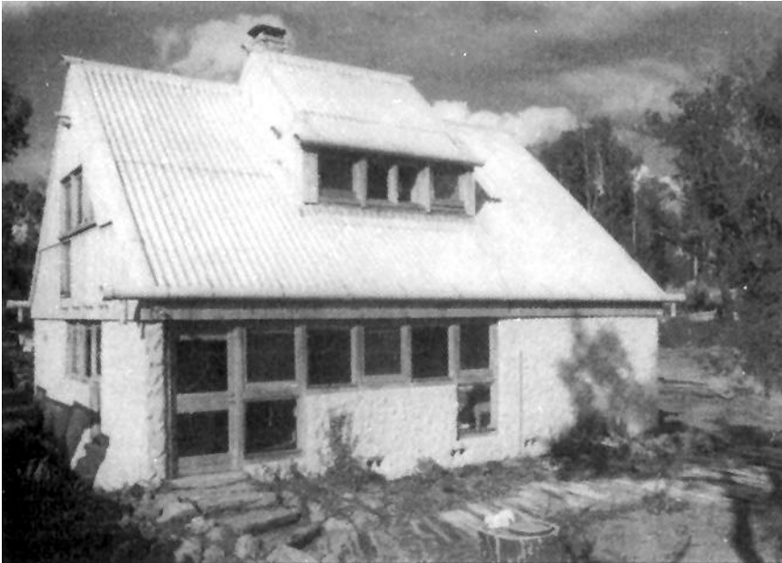
Loft homes have been built of a variety of different materials. This three bedroom home is made of pisé (rammed earth) and cost only $15,000 to build.
