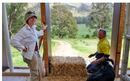
↑ Narelle and Rolf placing the first bale on the west wall.
