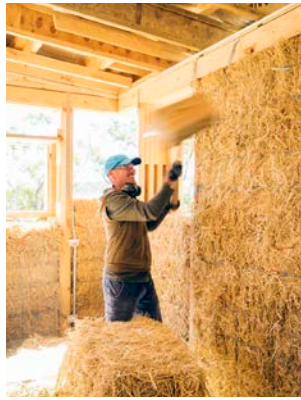
↑ Hands-on learning: straightening strawbale walls with 'Thor's hammer'; filling holes in walls with cob and learning to render.
