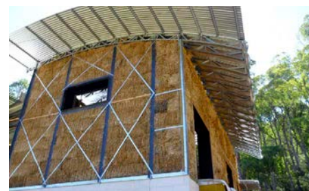
↑ The west wall ready to be rendered. The construction uses standard structural framing with bales as infill.
