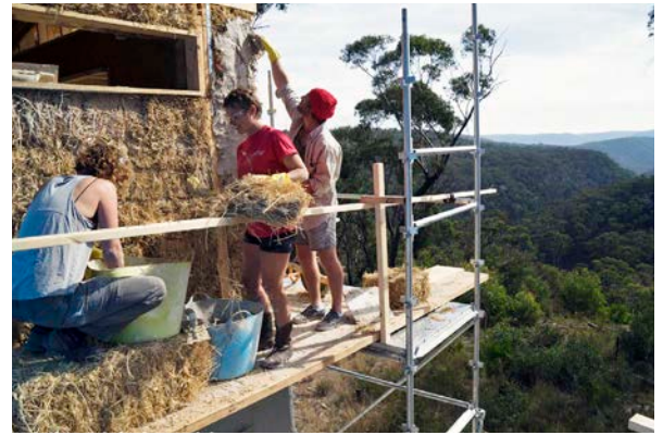
↑ Hands-on learning: straightening strawbale walls with 'Thor's hammer'; filling holes in walls with cob and learning to render.
