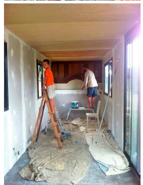
↑ → Construction commences in earnest: a roof is added (above), recycled from a rundown carport, window and door holes are cut, an internal frame added, windows installed (top right), insulation added, and plasterboard applied and then painted (bottom right).
