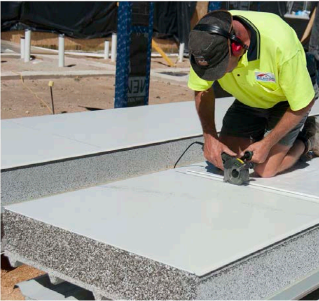
↑ Avoiding thermal bridges in the roofing panels—roofer pictured inserting sawcut gap between internal ceiling and external soffit to obstruct passage for heat conduction.
