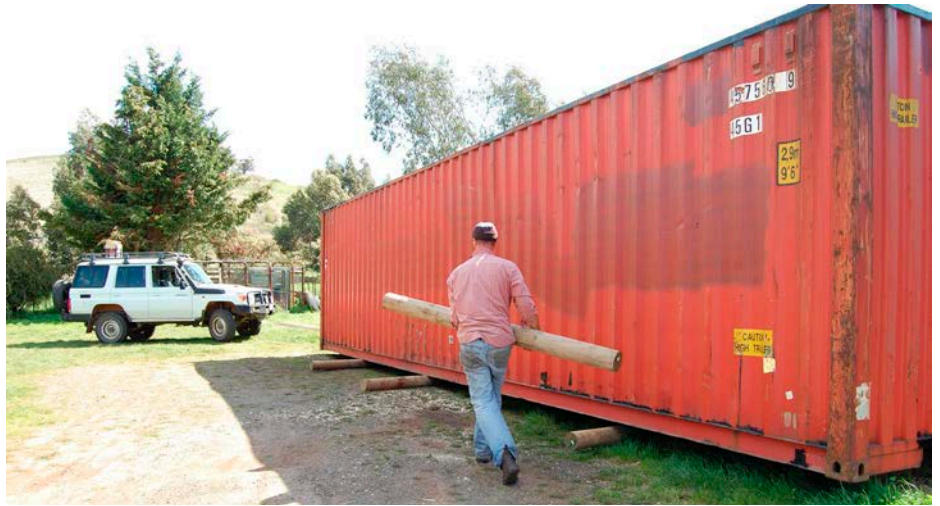
↑ Cranes weren't needed to move the container into position when they returned from holidays. They used fencing posts and a 4WD to shift the container about 50 metres and 90 degrees (to orient it for passive solar).
