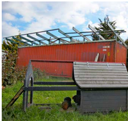
↑ → Construction commences in earnest: a roof is added (above), recycled from a rundown carport, window and door holes are cut, an internal frame added, windows installed (top right), insulation added, and plasterboard applied and then painted (bottom right).
