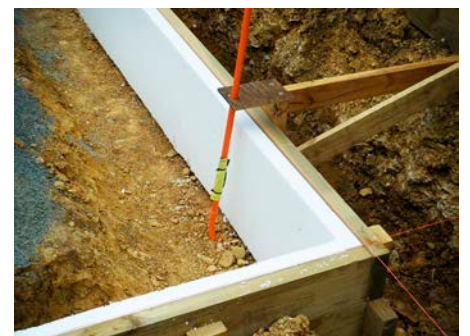
↑ The slab insulation, before pouring of the slab.
