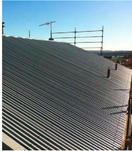
↑ The durability of materials subject to wear and tear, such as roofs and external cladding, is one consideration in designing a building to last. Colorbond Ultra comes with a 25-year warranty even in a coastal environment. Zinc cladding can be maintenance-free for 60+ years.
