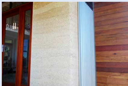
↑ Hemp-lime wall prior to rendering.
