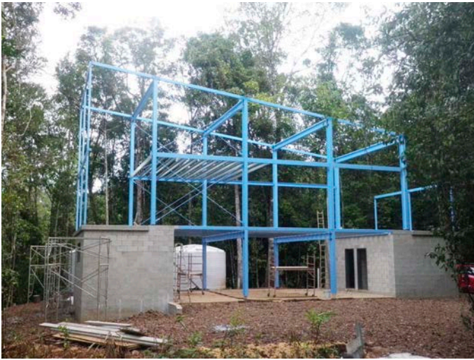
↑ Steel frame construction on top of the concrete block pods.
