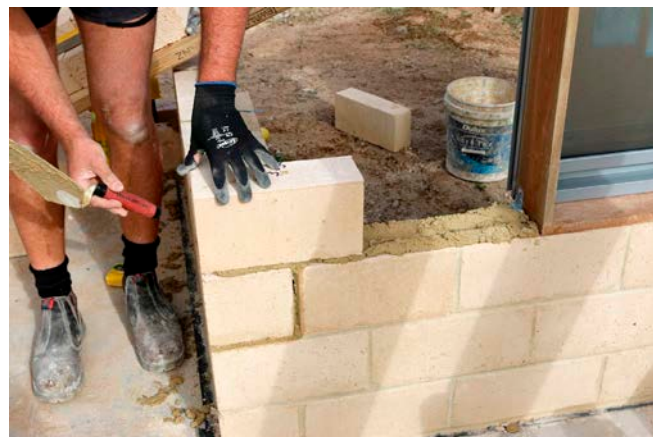
↑ Timbercrete uses wood waste to reduce weight and increase thermal performance compared to concrete, as well as to lock up carbon.
