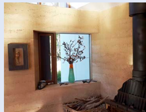
↑ The massive walls combined with insulation make for thermally stable and beautiful homes in even the coldest climates.
