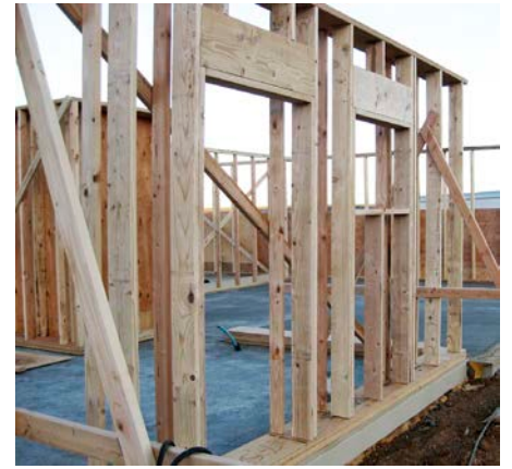
↑ Double stud walls allow for thicker wall insulation, ideal for colder climates.
