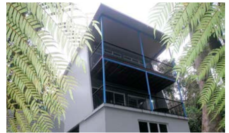
↑ Studio Nimbus: built to last in one of Australia's most beautiful, and challenging, regions. Page 54.
