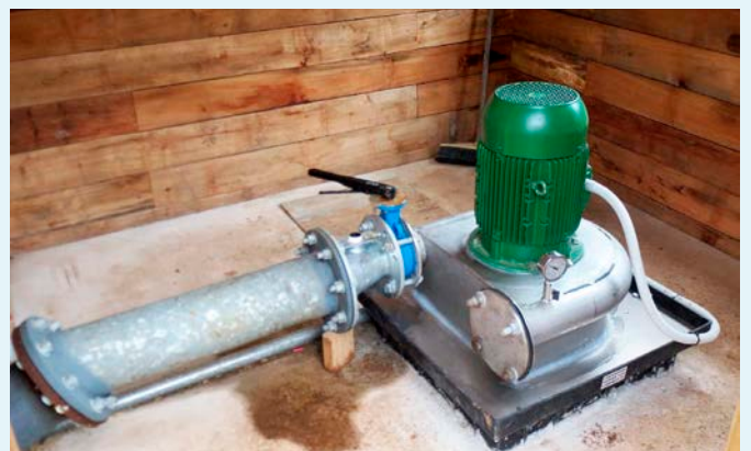
↑ The 7.5kW Platypus Power micro-hydro turbine.
