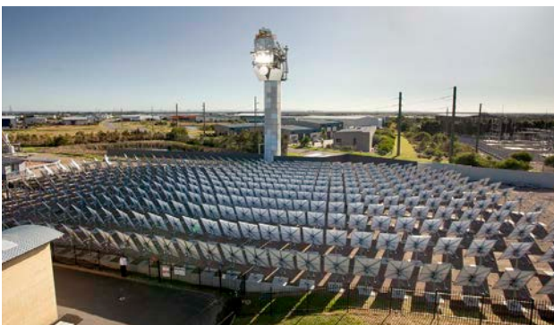
← Solar Tower 2 in operation at the CSIRO Energy Centre in Newcastle. CSIRO has used solar energy to generate hot and pressurised 'supercritical' steam at the highest temperatures ever achieved outside of using fossil fuels. www.bit.ly/1kw4A49
