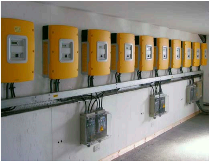
↑ The microgrid on the Isle of Eigg uses a bank of 12 SMA Sunny Island 5048 off-grid inverters and a Rolls 212 kWh, 48V battery bank for storage.
