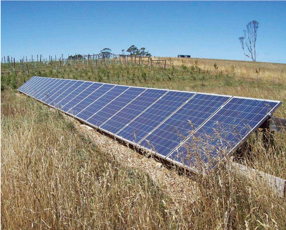
↑ The farm's large solar array (5kW) provides the electricity needs of the farm and tractor.
