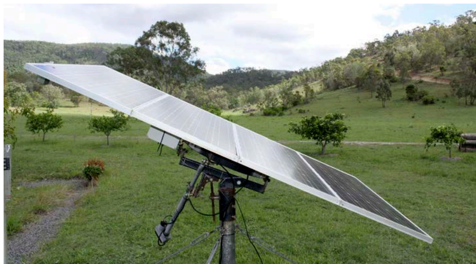
↑ 'Noddy' with four 80W panels tracking the sun.
