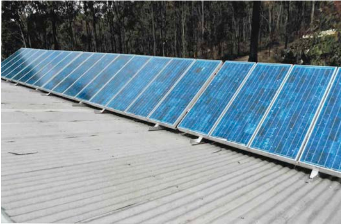
↑ Electricity comes from a solar array, with a generator for backup. Twenty 11-year-old 80W Solarex panels are mounted on the shed. An underground line takes power to the house about 70 metres away.
