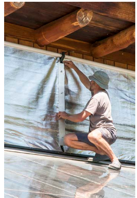
↑ Clerestory window blind end-joiner. Wind is the nemesis of lightweight materials. Here I am attaching a plate of aluminium to join the two blind edges together, clamping them against the window frame to keep out wind and embers.
