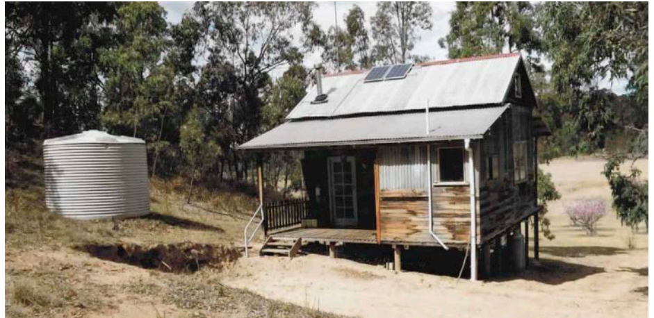
↑ This cabin was their home prior to building the RAL house, and has its own water (including hot water), flush toilet and electricity supply from two 80W panels and six 2V gel batteries. It's now used by guests and family.
