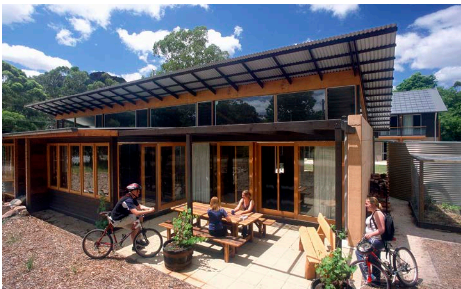
↑ Eco doesn't need to be expensive. The Grampians Eco YHA in Victoria was specifically designed with the aim to use 50% less energy and water than conventional hostels. It includes solar PV tiles incorporated in the roof.
