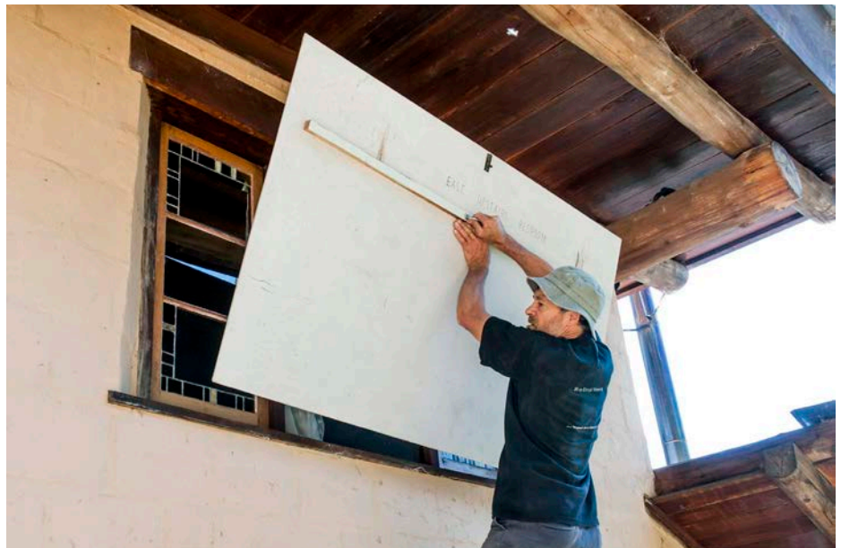
↑ Standing on the ladder, placing the cement sheet over the bedroom window. I use an assortment of heat shielding; this one is perhaps the most awkward.
