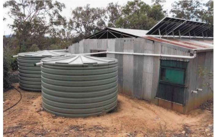
↑ Water is gathered from the shed and house roofs, and stored in six 5000 gallon tanks. That's 30,000 gallons, or 136,500 litres! Batteries sit behind the shade cloth on the western wall of the shed; note the two external vents from the battery box at the back of shed.
