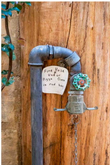
← Valve assembly for a fire hose. Standpipes for fire hoses need to be suitably sized, and hoses easy to find.
