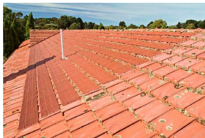
↑ Solar pool heating collectors are simpler than solar water heating units, consisting of grids of rubber pipes. This unit, from Sunbather, is the same colour as the roof to make it less conspicuous.
