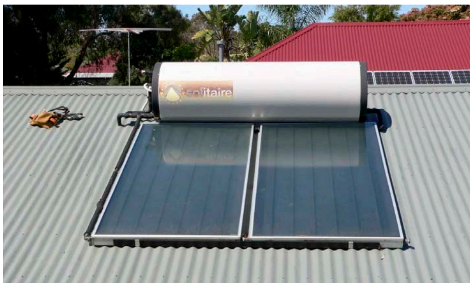
↑ The well-studied solar hot water system.
