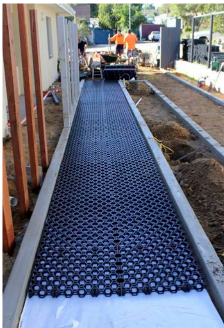
↑ Laying the Nero Drainage Cell to create an even surface that will drain excess water.
