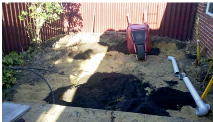
↑ Addition of topsoil and bentonite clay soil amendment to the excavated plot.
