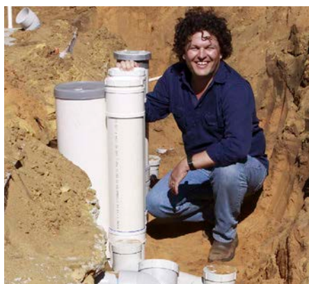
↑ Josh Byrne installs the Grey Flow greywater system in Josh's House. Page 28.
