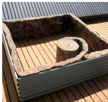
↑ The garden beds under construction. They were first insulated with a 75 mm layer of rockwool and sealed from the soil and weather with a tarpaulin. The drainage pipe can also be seen in the top photo.
