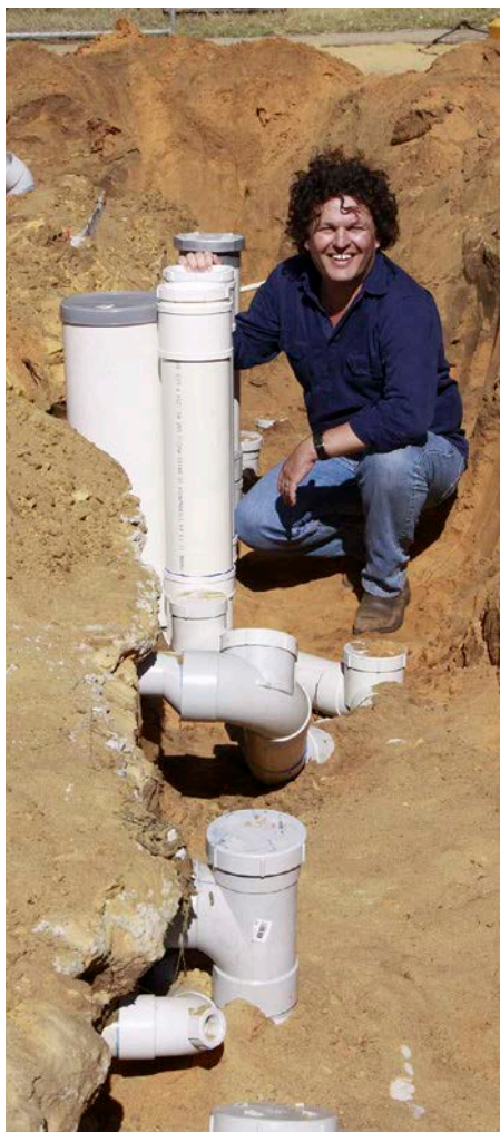
↑ The Grey Flow builder’s kit greywater system is mostly underground.
