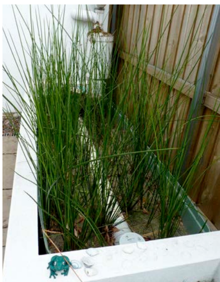
↑ This reed bed treats greywater before final sterilisation in a Sydney suburban garden. Page 36.
