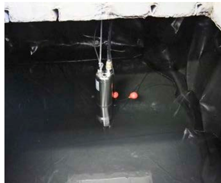
↑ The submersible pump is located inside the underground rainwater tank.
