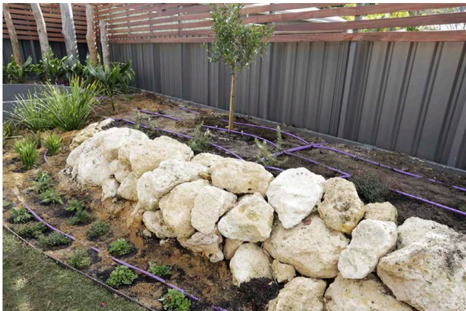
↑ Greywater is fed to the garden via a series of drip-feed lines. Here they can be seen before being covered in 100mm of mulch.
