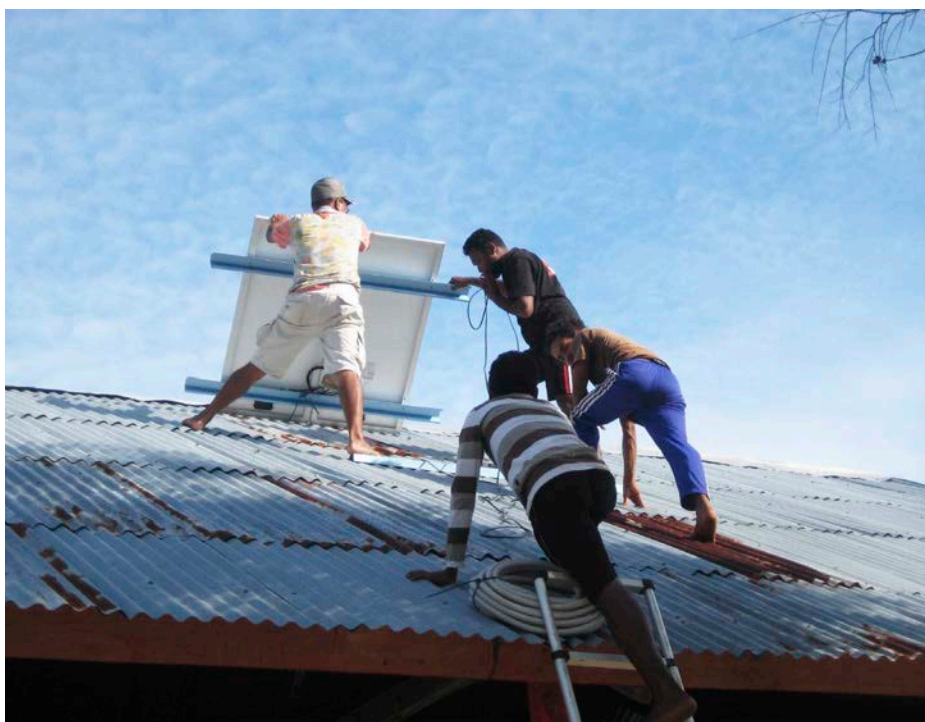
↑ Installing the panels on the school roof.
