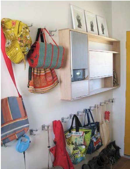
↑ The PV system monitor is built-in—in a cupboard in the entry hall—with the hooks below it reused from the portable classrooms. The 2kW PV system is generating around 10–14kWh in October, against usage of about 5–6kWh for this all-electric house (usage will be higher in winter with heater use).
