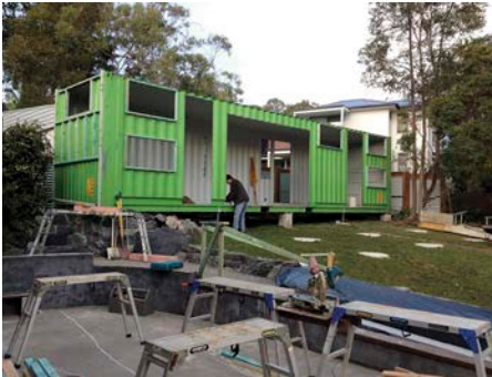
↑ Karina and Tony Rothacker's two-bedroom container unit (above). At left, the container begins its transformation to a light-filled house with the holes cut out for doors and windows.
