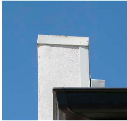
↑ The parapet cap sheds moisture away from the walls.
