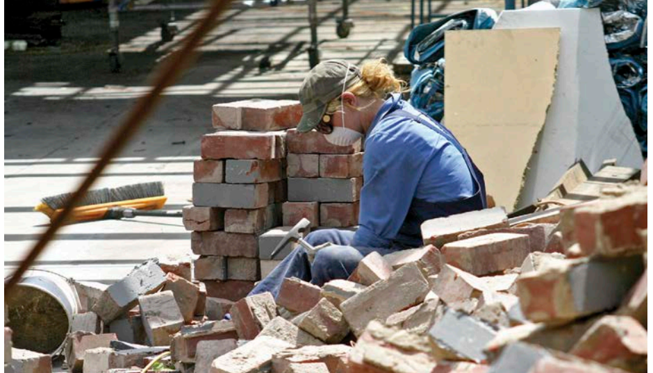
↑ Cleaning bricks for reuse at a Resource Work Cooperative deconstruction site.
