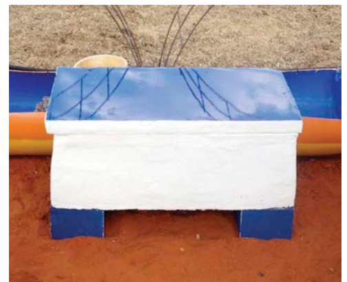
→ This papercrete worm farm doubles as a seat. The thick papercrete walls will support heavy loads as well as keeping the worms cool and healthy.
