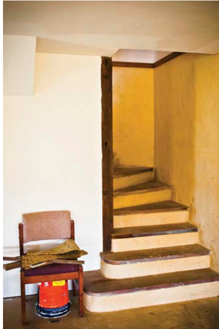
← Stair treads with rendered risers. Above: Peter's four-year-old, Turlough, in what will be the cellar/cool store.
