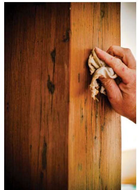
↑ Oiling a recycled timber internal post.
