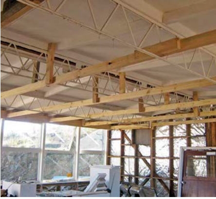
↑ Installing the false ceiling.
