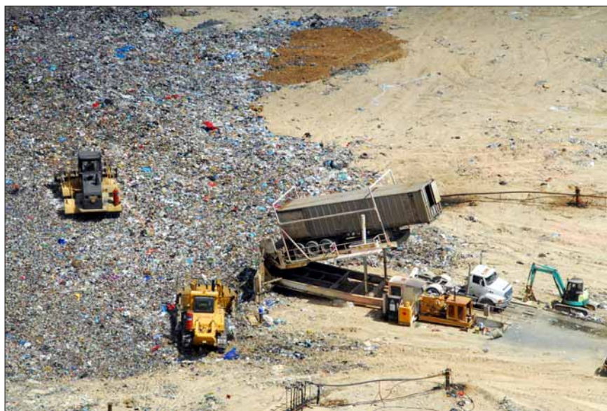
The containers are emptied and then bulldozers spread and compact the garbage.
