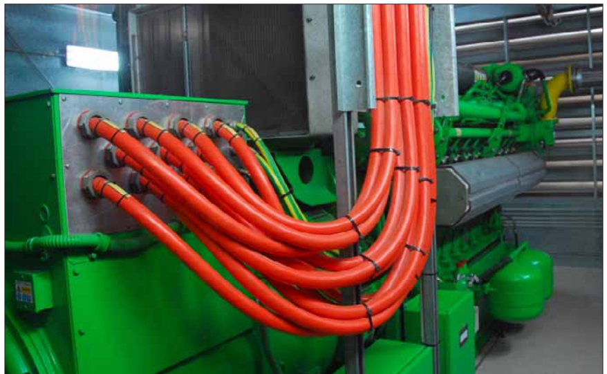
Top: Boring machines drill wells in the garbage that has now reached a thickness of 60 metres. These wells are used to recirculate leachate and collect methane gas. Below: The methane is cleaned and then burnt within three 1.1MW Jenbacher 20 cylinder engine/generators. The electricity is then fed into the national grid.
