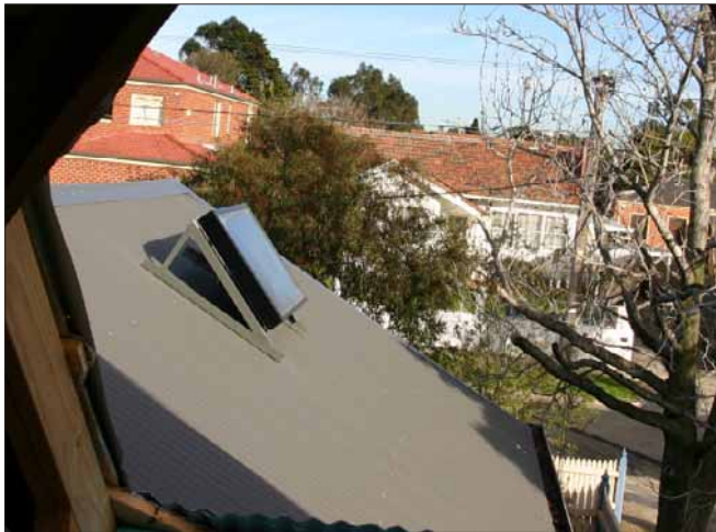
Shane's rental property retrofits (clockwise): the old and breezy non-insulated tile roof being removed to install aircell insulation and batts; bathroom walls packed with insulation; one of the downpipe diverters which waters the garden with rainwater; the roof-top SolarVenti warms and circulates air in the front of the house during winter.
