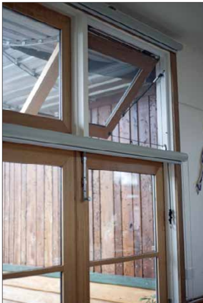
Operable windows with the old pier external cladding in the background.
