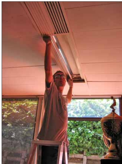
Left: Damien Moyses reinstalls a fluorescent tube with a new reflector to improve lighting levels. Right: Simon Wilson and the new water saving tap for the kitchen.
