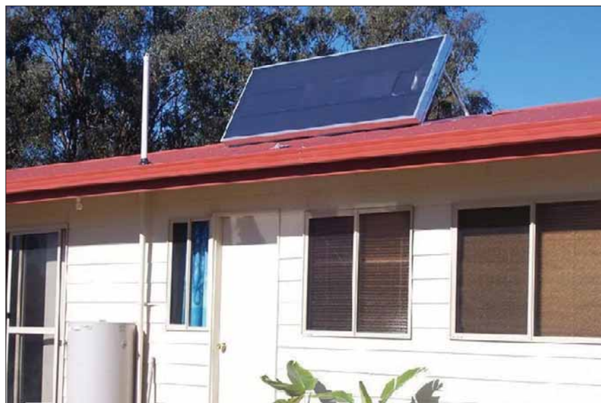
Solar collector ventilators like the Solar Venti can help exhaust hot air and also work in the cooler months as air warmers.
