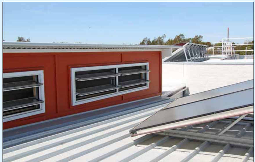
Electrically controlled double glazed louvre highlight windows with a rooftop solar water heater, and a PV array in the distance on an adjoining house.
