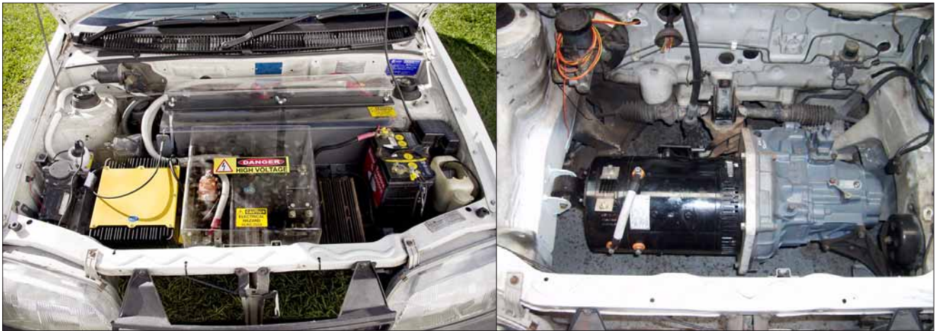
Under the bonnet: the yellow box on the left is the speed controller. The contactors and other gear are under the transparent cover in the middle and the auxiliary 12 volt battery is on the right. Two more batteries are at the back and the motor is underneath all of these components (right).
