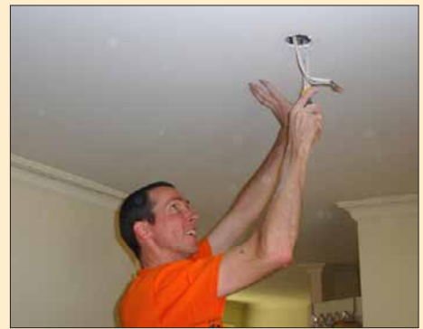
Don Batson replaced halogen downlights with energy efficient LEDs at his investment property, as shown in ReNew 111 .
