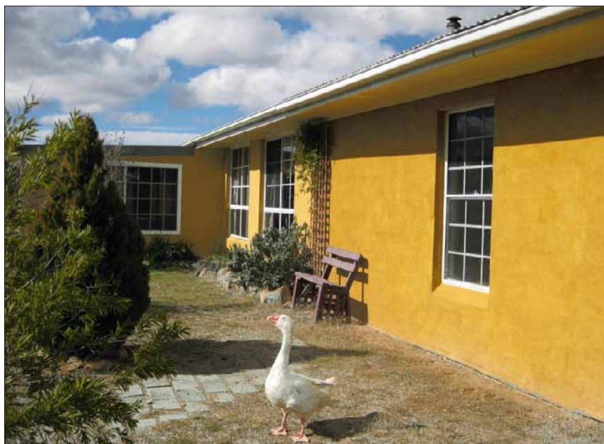
A big goose plus big 600mm eaves on the north-facing side of house let winter sun in, and keep the summer sun out.
