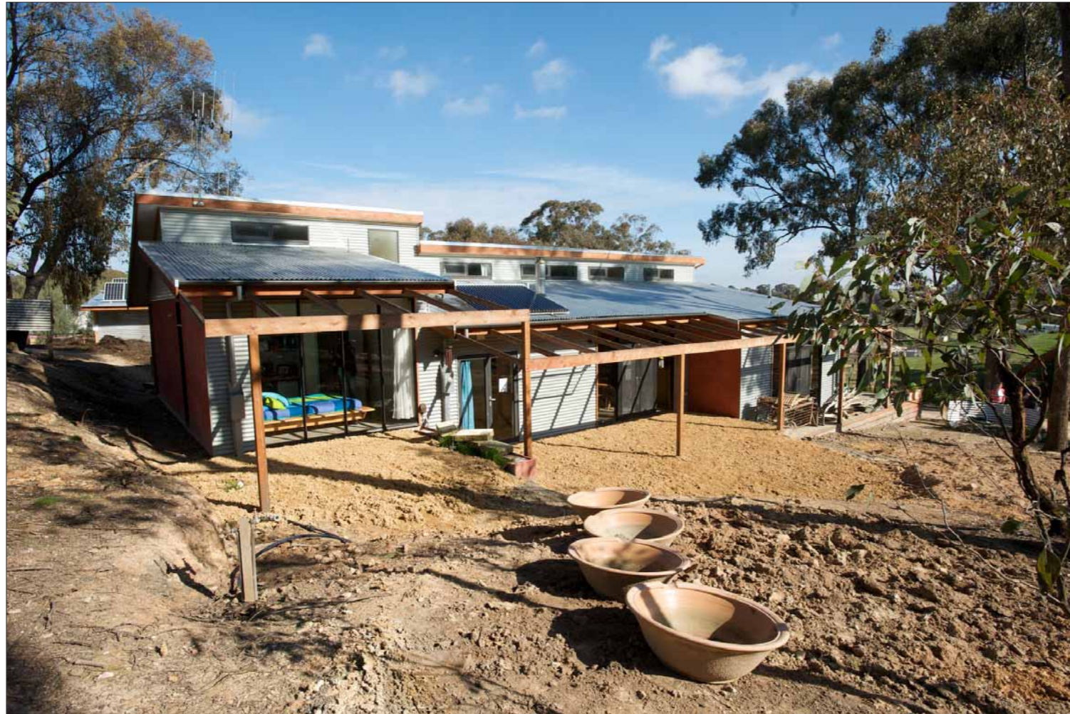
Clockwise from top: Lot 4 at Murrnong is constructed from lime-rendered strawbale, lime-rendered concrete blockwork and colorbond sheeting. Colorbond windspray (light grey) has been used on the external walls for heat reflective qualities; Inside lot 4 clerestory windows bring in natural light; Clever use of space with loft spaces in the kids bedrooms thanks to a 4.5 metre ceiling.
