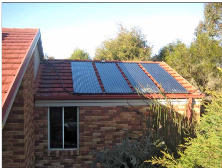
The house today still has the four solar hot water panels which are attached at the start of winter. Below: The house as it appeared in ReNew 77.
