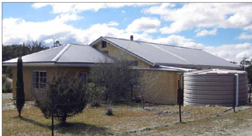
The three rainwater tanks have a combined 42,000 litre capacity.
