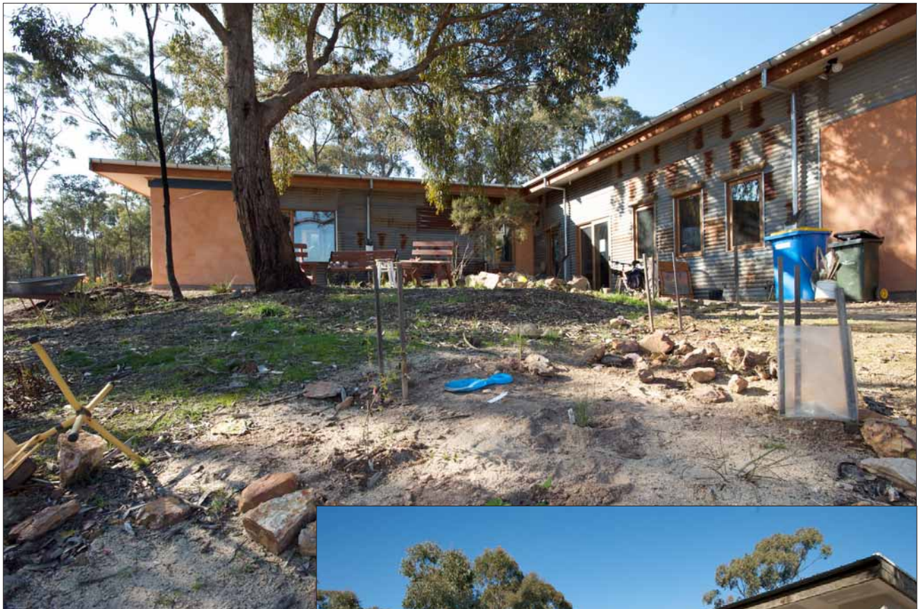
Top: Lot 2 at Murrnong is strawbale construction featuring a greenhouse to the northern front of the home. The greenhouse opens to the rest of the house, providing a form of passive heating on cold winter days and a place to grow produce in the cooler months. Right: This home featured in ReNew 110 for its buried pipe cooling, or earth tubes system, and is made from double skin concrete block walls with an insulated air cavity and lime render.
