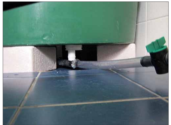
Clockwise from top left: The ring used for the outlet hole; The barbed shank assembled ready to be pushed up into the bucket. The hose with the green in-line tap connects to the pump inlet and the other short hose ends with a black tap that is normally kept closed; eight aerated concrete blocks support the bucket. They are covered in gutter silicone so they don't absorb water and grow mould; the pot scourer next to the outlet sits neatly in the hole to act as a filter, primarily for hair.
