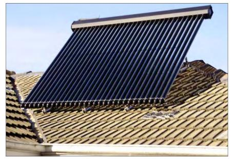
Active solar water heaters have the advantage that only the collector is on the roof.
