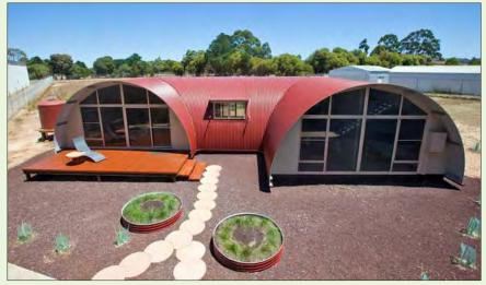
ferent components to create their own individual living space with all kits having standard safety and building features. They use mostly plantation timber and other renewable and recyclable components in construction, meaning the energy used for production is lower than other buildings of similar dimensions
