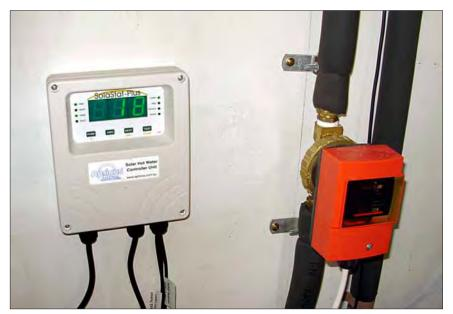
Active systems have the disadvantage of added complexity due to the need for pumps, controllers and temperature sensors, thus increasing the likelihood of problems.
