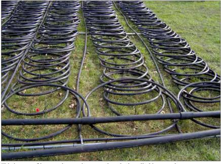
This is a set of heat exchanger loops ready to be installed in a pond.
