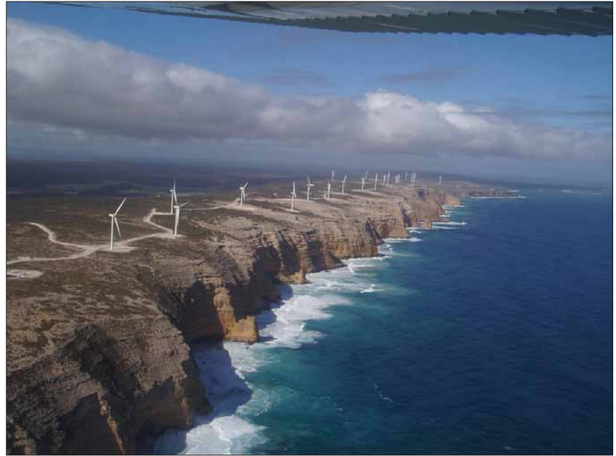
Photo by Richard Pocknee, Project Manager, Cathedral Rocks Wind Farm, SA.
