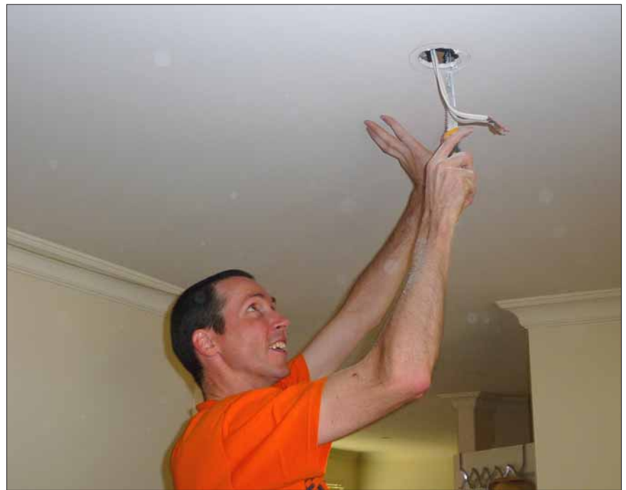
A quick cut with a plasterboard saw and the new light fittings can go straight in.
