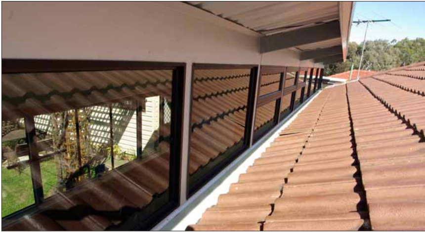
North facing windows and eaves letting natural light in.
