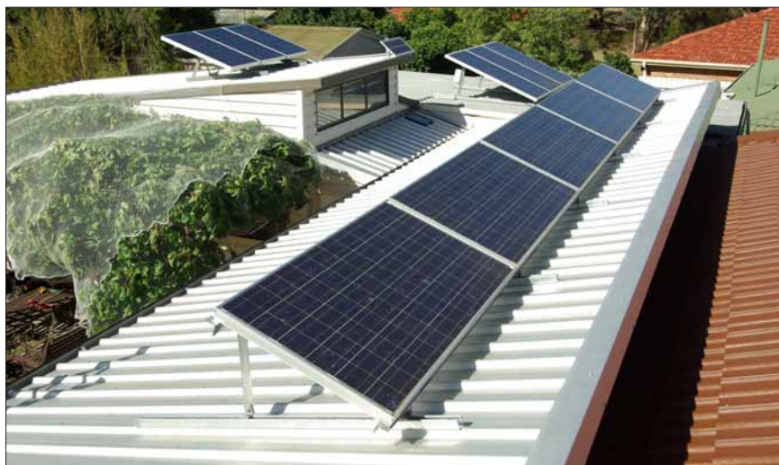
A 1.5kW photovoltaic system, with a smaller 240 watt system in the background.
