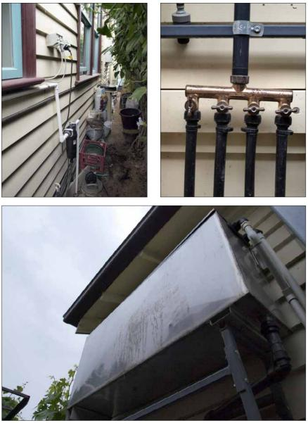
Clockwise from left: The pump with the sump in the ground to the right; the four line manifold that distributes water to different parts of the garden; the stainless steel header tank made from recycled materials.
