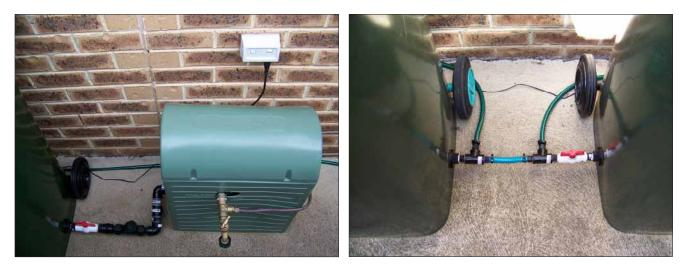
The rainwater can be sent to the washing machine and hot water service via the RainBank pump. Right: Connections and isolation valves between the tanks.
