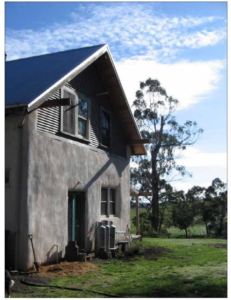
The walls have been rendered with a lime and sand mix up to a 50mm thick layer.
