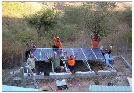
Hands up for solar: seven 130 watt solar modules power the pump in Oecussi.
