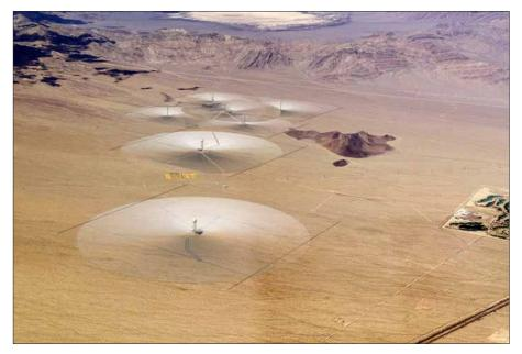
project. This involves thousands of sun-tracking mirrors (heliostats) that focus sunlight onto a central tower, which contains a boiler. The water therein is heated to around 550°C, producing high pressure steam that drives a standard steam turbine that turns a generator.
