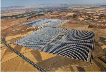
has two vast energy storage tanks which each hold 28,500 tonnes of liquid salt, so the plant can generate electricity day and night. A full thermal storage can provide power for 7.5 hours at maximum load.
