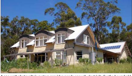
A 920 watt photovoltaic system provides nearly enough electricity for the household.
