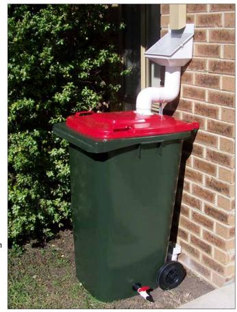
up as an all-in-one unit in its own weatherproof polyethylene housing and cover.
