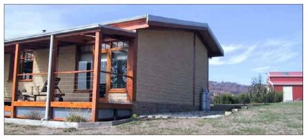
This well finished earth brick house survived the fires when the owners and a friend defended the property. Flames were reported to be two to three times the height of the surrounding forest area. The site is located on a ridge with the slope away from it on both sides. This photo indicates the quality workmanship and the sealing off of the timber where it passes through the wall, preventing embers entering the roof space.
