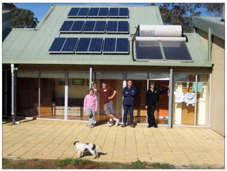
Can state governments support more families like this? The Packer family is leading the way when it comes to living sustainably. Household hot water is from the roof mounted solar collectors and storage tank, with a gas boost unit for the cooler months. The 144oW photovoltaic system supplies around half of the electricity needs for the family of five.
