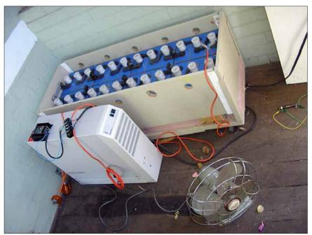
The UPS solar power system in the testing phase (hence the wiring spaghetti). Discarded devices like this make ideal inverters in smaller systems. The fan is a test load. The white box is the UPS, the PL20 is sitting on top of it and needs to be mounted vertically for cooling. The battery bank is shown behind with the lid of the battery box removed. It has large holes in the sides to prevent hydrogen gas build up in the box.
