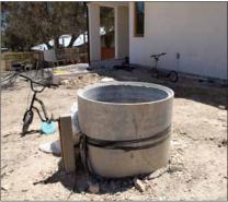
Top: This house has two 225mm wide concrete pipes underneath as part of an earth tube system. Bottom: The upstand which buffers the earth tubes from unwanted wind-driven air.
