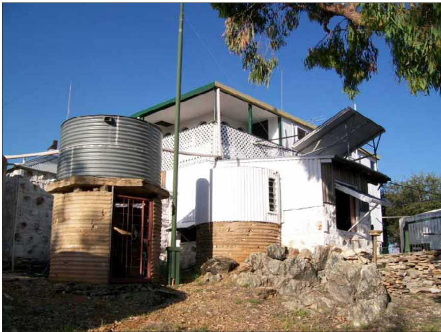
Eric Foulke's shed is made from home made concrete bricks and and recycled timber.
