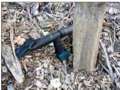
6. One inch poly, one inch poly T, and an end stop using a cable tie.
