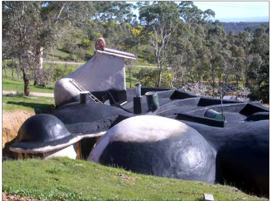
Top left: it was all concrete blocks to start with. Bottom left: steel reinforcing added strength to the roof. Right: It's all in the load-bearing domes when it comes to earth-covered structures.
