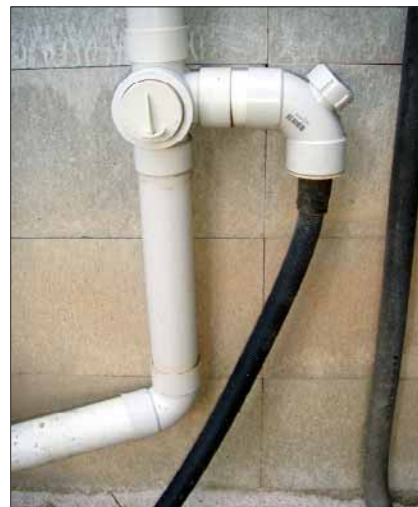
2. The diversion valve. When I have too much rain and the trees don't need watering, I turn the valve and the greywater goes back into the sewer. I used 25mm corrugated greywater pipe to get to the trees.
