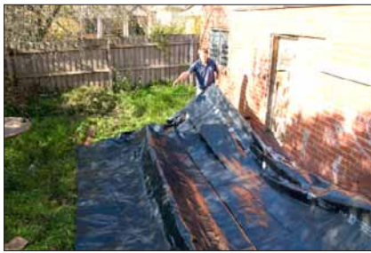
4. Put down the concrete underlay.
