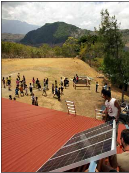
Fixing the solar panels with the help of teachers in Nanutana.
