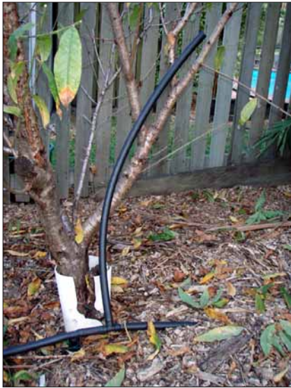
4. The first tree also has a 1.3 metre overflow pipe. If there is a blockage lower further down the pipe, or too much flow, it simply comes out here. This is below the level of the house. Make sure yours is too.
