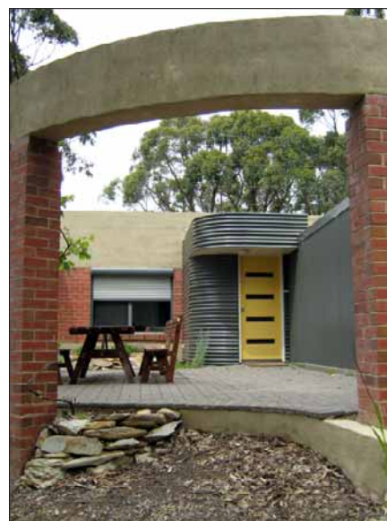
Paul’s earth-covered house with the protective spark-arresting air-lock at the entrance and co-ordinated designed roller shutters on the windows. These features make the house virtually bushfire proof.
