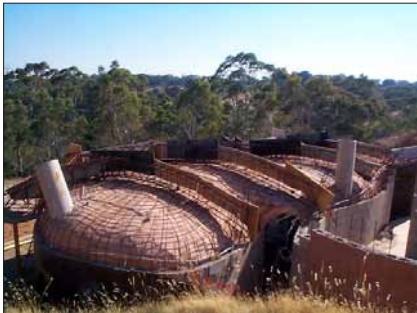
Top left: it was all concrete blocks to start with. Bottom left: steel reinforcing added strength to the roof. Right: It's all in the load-bearing domes when it comes to earth-covered structures.
