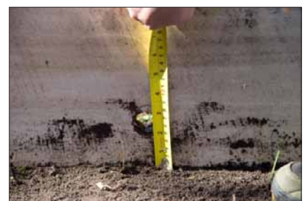
3. Drill a hole 5cm from the bottom to allow excess water out.
