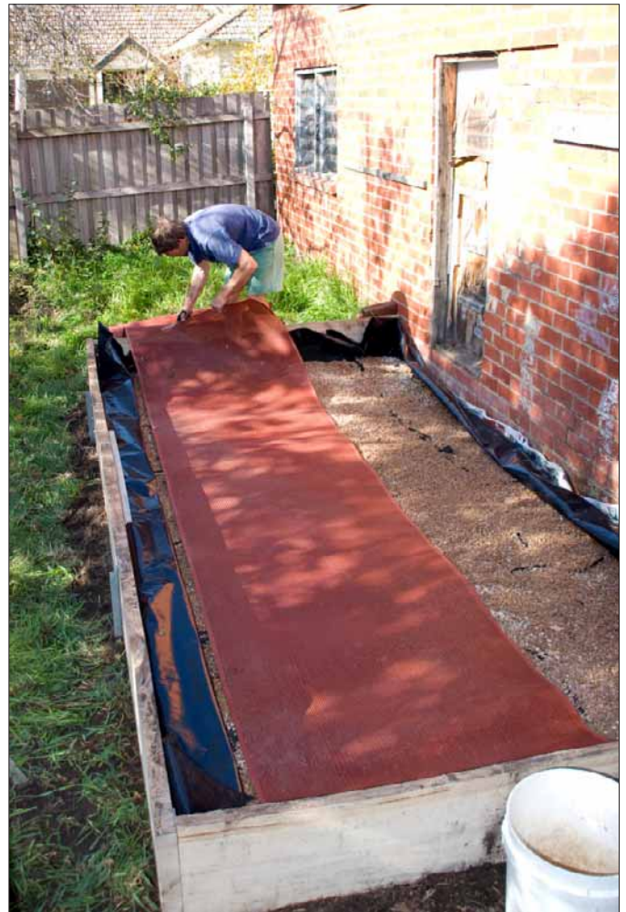
7. Shade cloth, used as a highly permeable water distribution layer.
