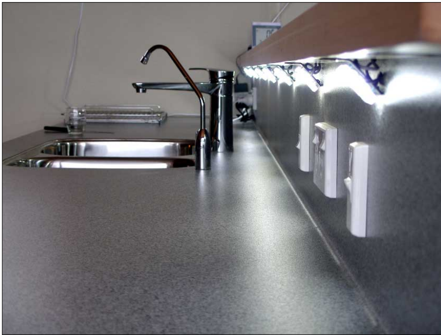
The kitchen bench lit with seven 1 watt LEDs. All the LED mounting hardware and accompanying power supplies were constructed by Michael because no stock items were available at the time of construction.
