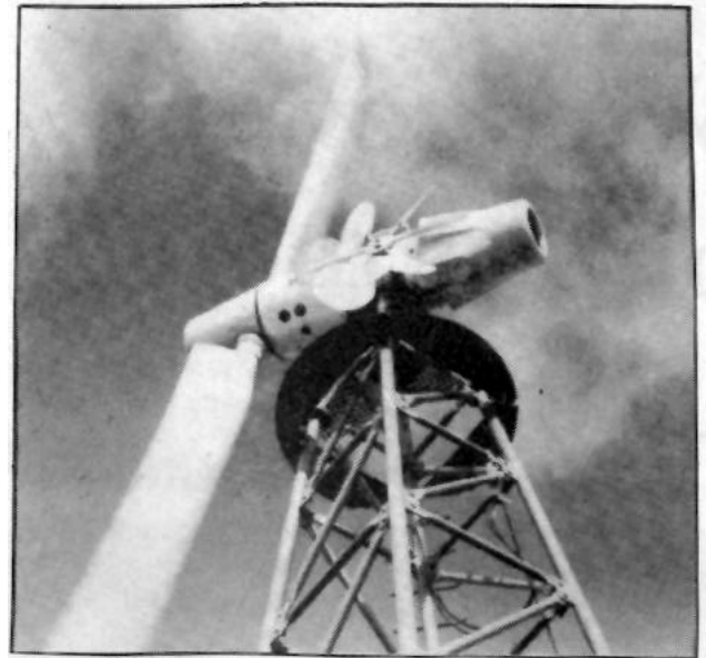
The MAN generator was manufactured in West Germany
