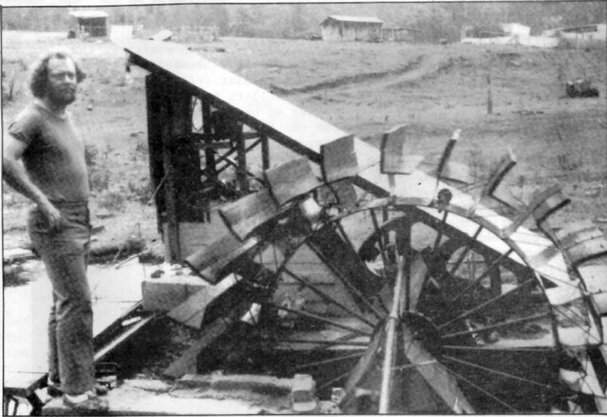
Lawrie Lang stands on the dam wall near his water wheel.
