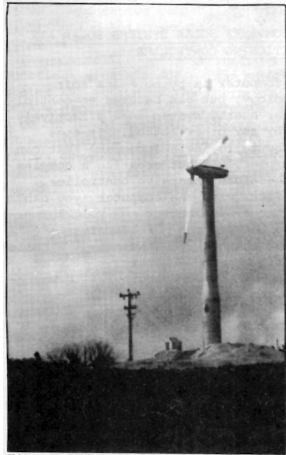
The Nordtank has two generators for its two speeds, a 15 KVA and a 75 KVA.
