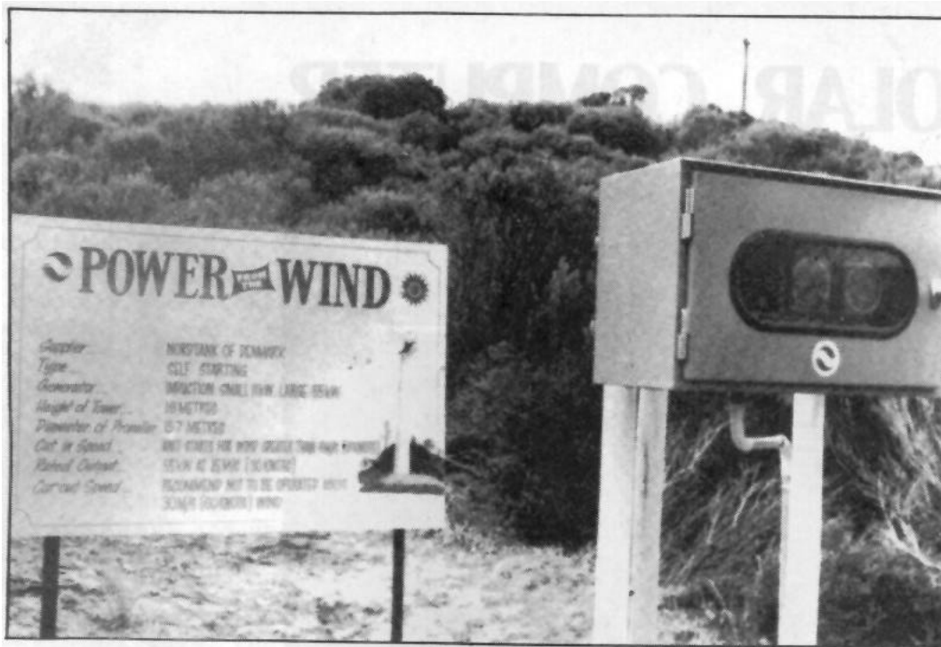
The information board and output monitoring board for the "Nordtank" wind turbine.
